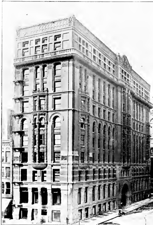
PHENIX INSURANCE BUILDING. Supplied with Hale Elevators.
