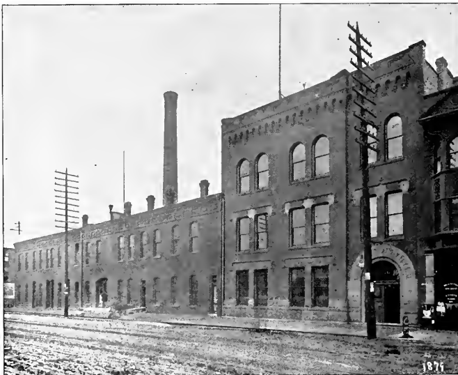
MAIN POWER STATION, CHICAGO CITY R. R. COR. 20TH AND STATE STS.
