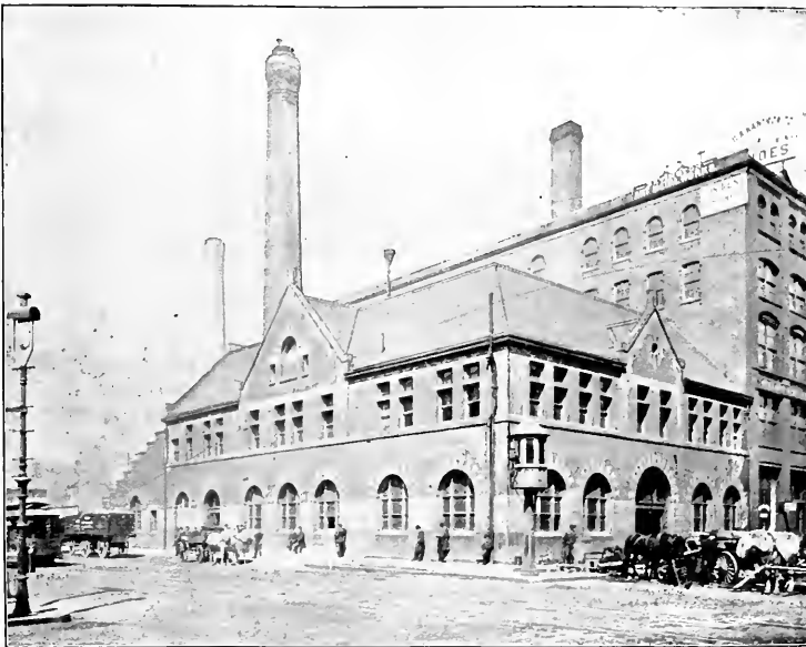
POWER HOUSE, WEST DIVISION STREET R. R., WASHINGTON AND S. JEFFERSON STS.
