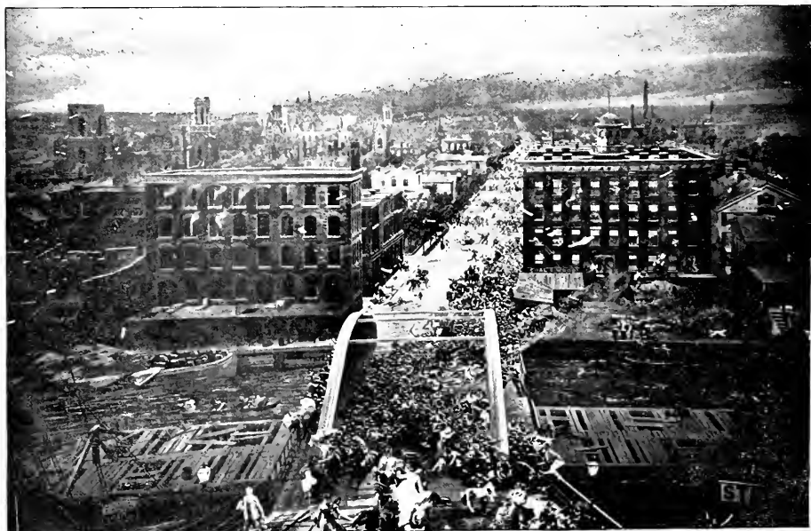
RUSH STREET BRIDGE, LOOKING NORTH.
