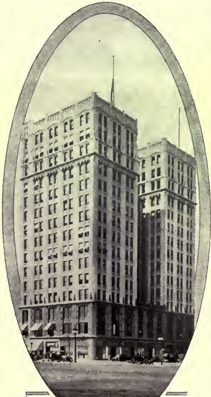
MICHIGAN BOULEVARD BUILDING Michigan Blvd. & Washington St., CHICAGO
