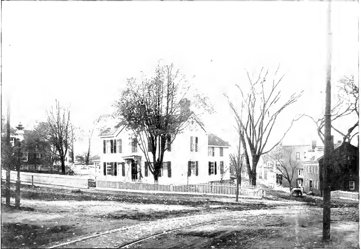
RESIDENCE OF EX-MAYOR GEORGE S. TAYLOR.
