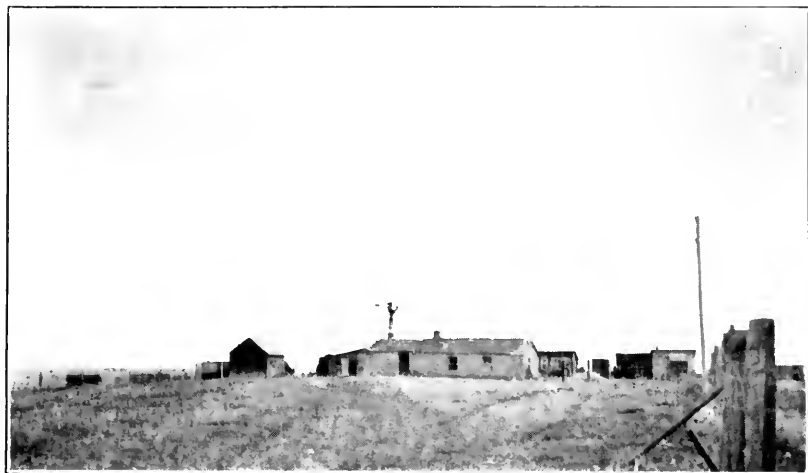
SOD HOUSES, STILL USED FOR DWELLINGS.
