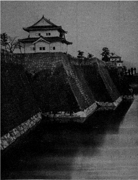
BATTER. —A castle in Japan, showing the batter, or backward slope, of the embankment walls.
