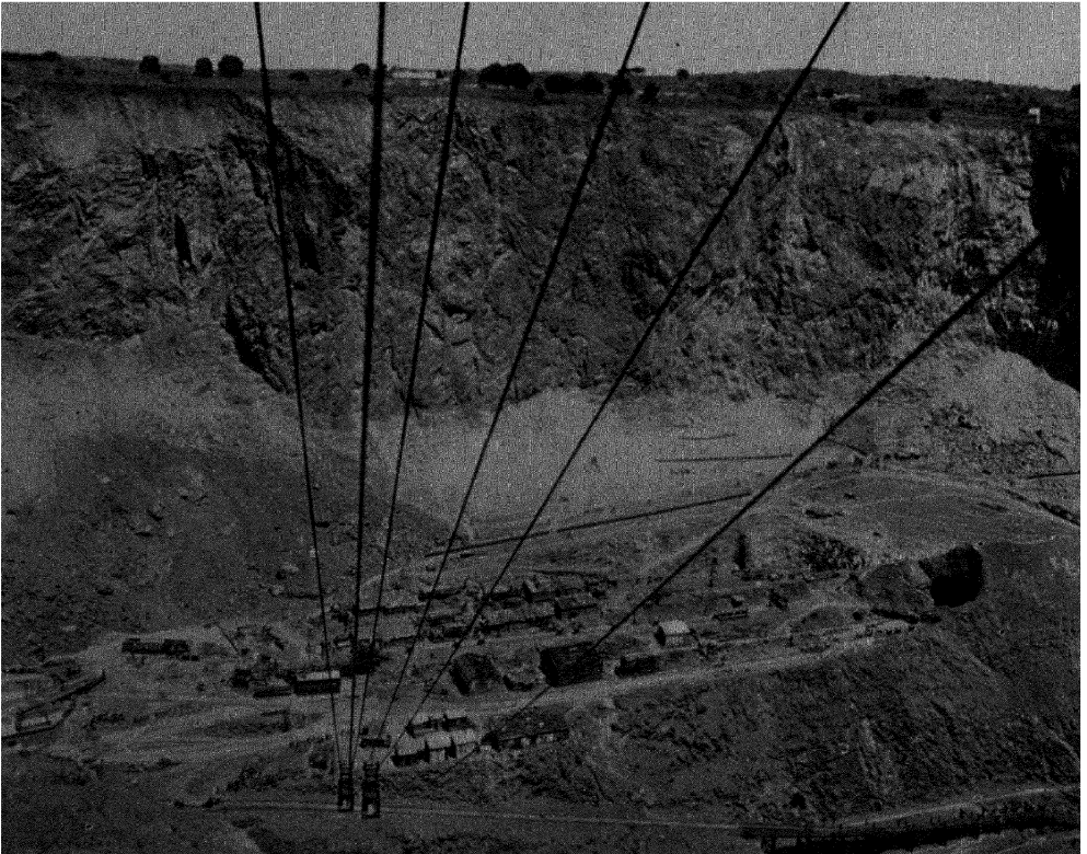
ROPEWAY. —An aerial rope on which men or materials can be transported is a ropeway. This picture shows the 1000-foot ropeway connecting the excavation of a Transvaal diamond mine with the surface.
