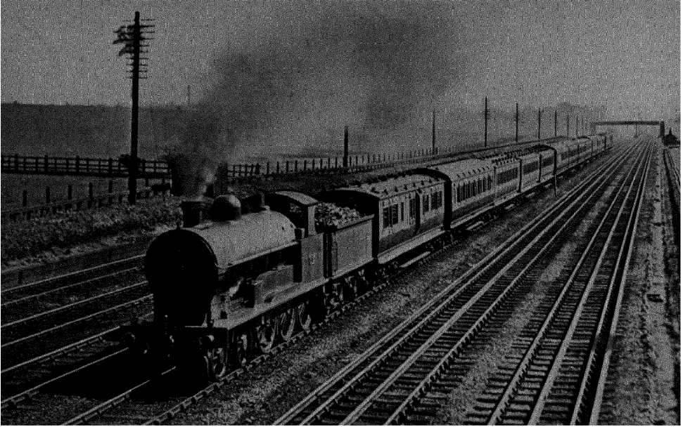
PERMANENT WAY. —The finished road-bed of a railway, with its tracks, bridges, signals, switches, etc., is the permanent way. This picture shows a section of a permanent way, with three pairs of roads. The two on the left are for steam trains and that on the right for electric trains.
