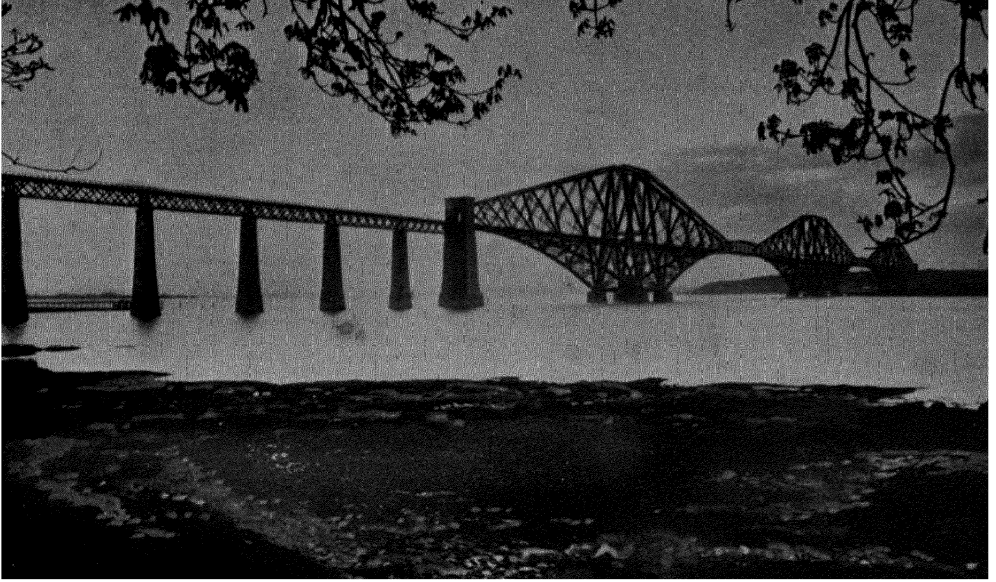
FIRTH. —In Scotland a narrow inlet or arm of the sea is called a firth. The Firth of Forth, shown here, is spanned by a cantilever bridge, with enormous spans and a total length of over a mile and a half. The Forth bridge is the largest cantilever bridge in the world. It carries a double railway track.
