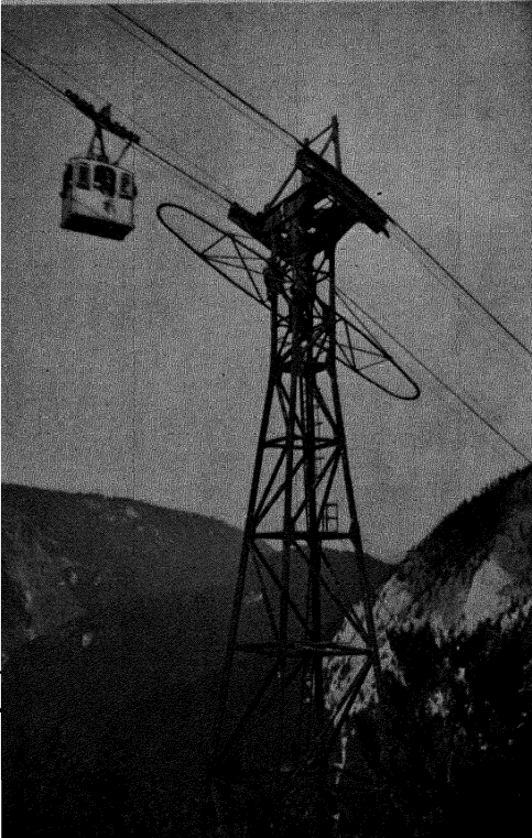
CABLE-WAY. —A wire cable carried on standards conveying a load across the Feuerkogel, Austria.
