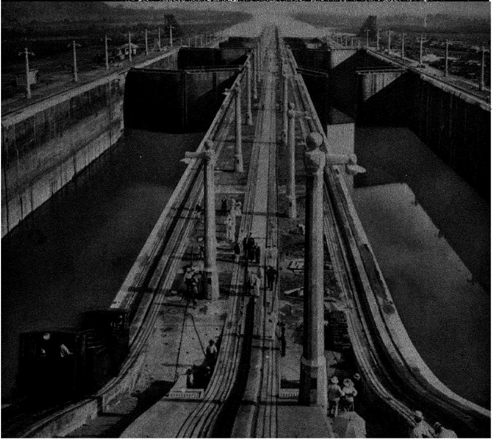
LOCK. —The Gatun Locks on the Panama Canal. Such locks provide a series of steps by which vessels are able to mount or descend from one level to another. The invention of the lock enabled canals to be cut through districts that were unlevel and hilly.
