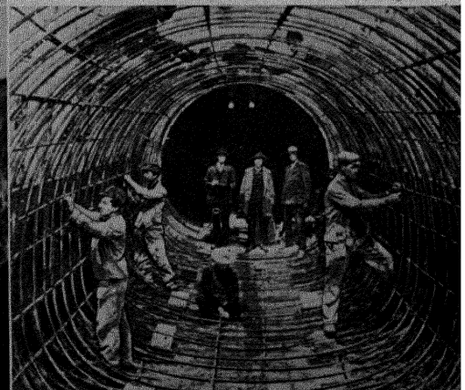
CULVERT. —Workmen repairing a culvert, or arched channel built under roads or canals to carry water.
