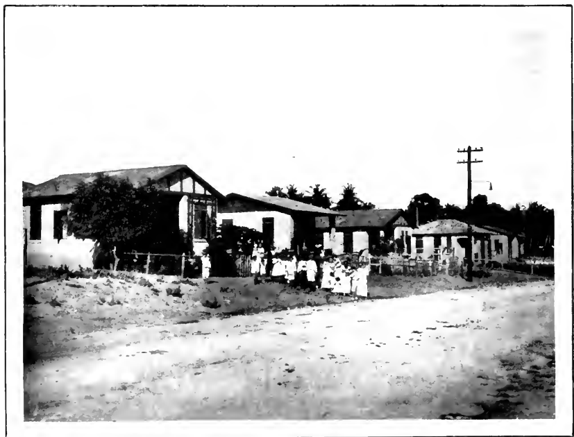
HOUSES BUILT BY THE MUNICIPALITY OF SAN JUAN AND SOLD ON LONG TERMS TO WORKINGMEN.
