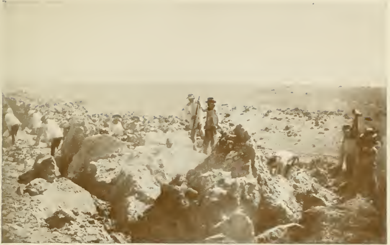
The Nitrate Pampa: Opening up Trench after Blasting.
