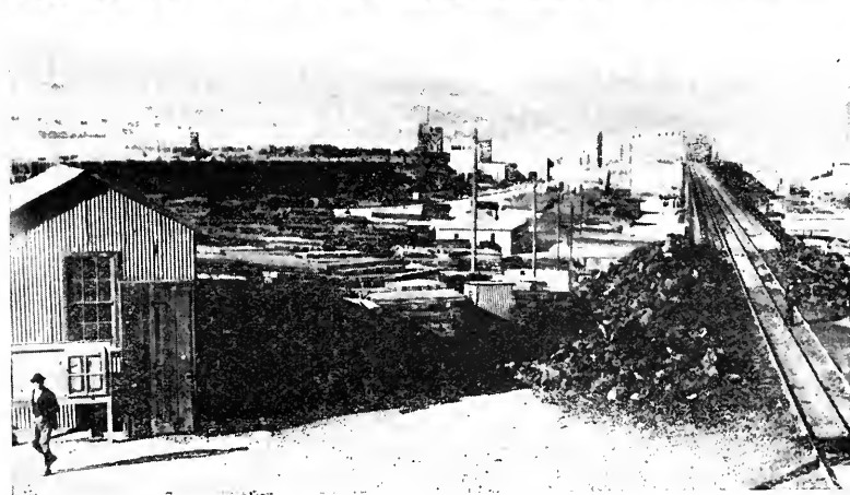
Curanilahue Coal Mine, Arauco Province. Dulcinea Copper Mine, Copiapó Province. Chuquicamata Copper Mine, Antofagasta Province.
