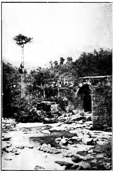
BRIDGE OVER GO-SHI RIVER.
