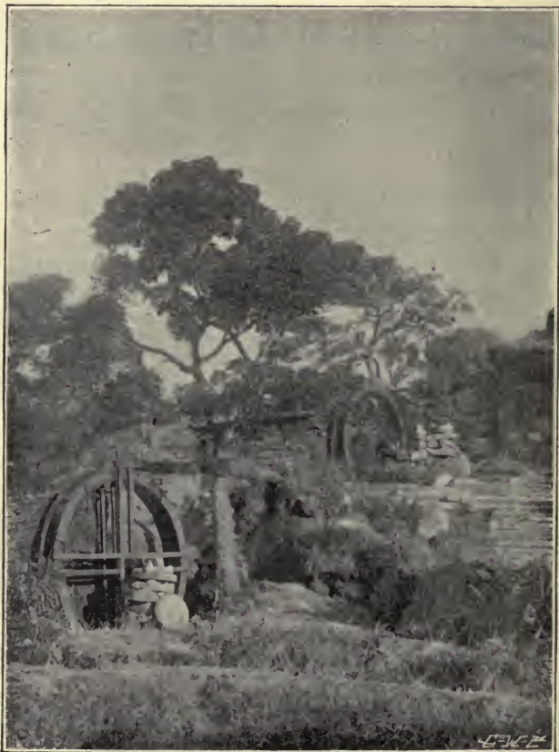
UNDER- AND OVER-SHOT WHEELS. (By permission of Messrs. Newton and Co.)
