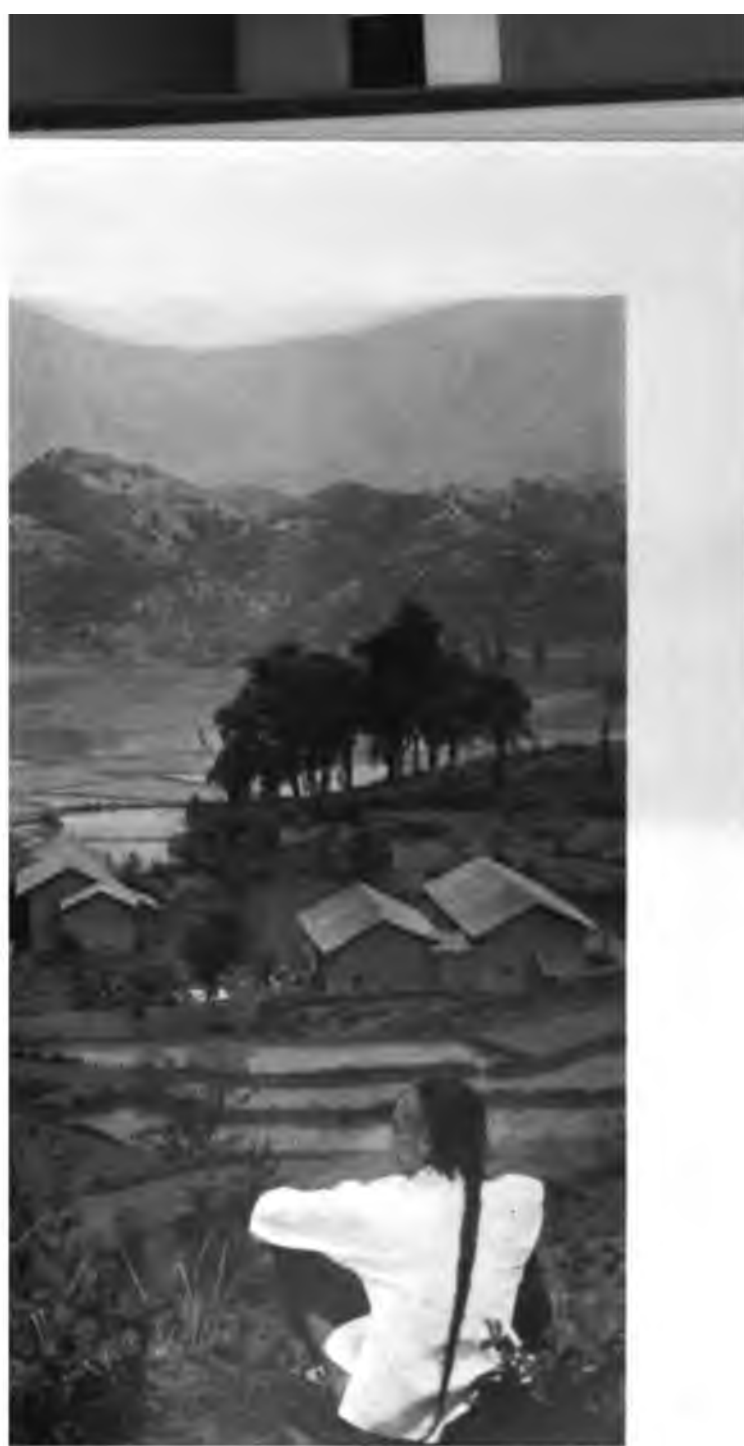
400 miles inland, tea district, Kiang-si province. Tea in foothills, rice (partly) fields in meadow. The in houses are erected by Russians to store tea.
