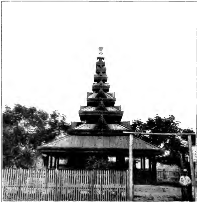
THE CHAPEL OF THE GOOD SHEPHERD, NEAR MANDALAY, BURMA, BUILT IN THE STYLE OF A BUDDHIST STUPA
