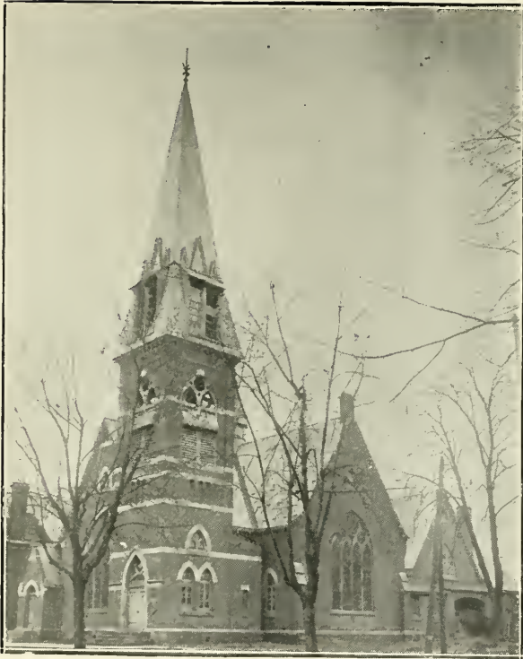
St. Peter's Lutheran Church, Middletown, Pa.
