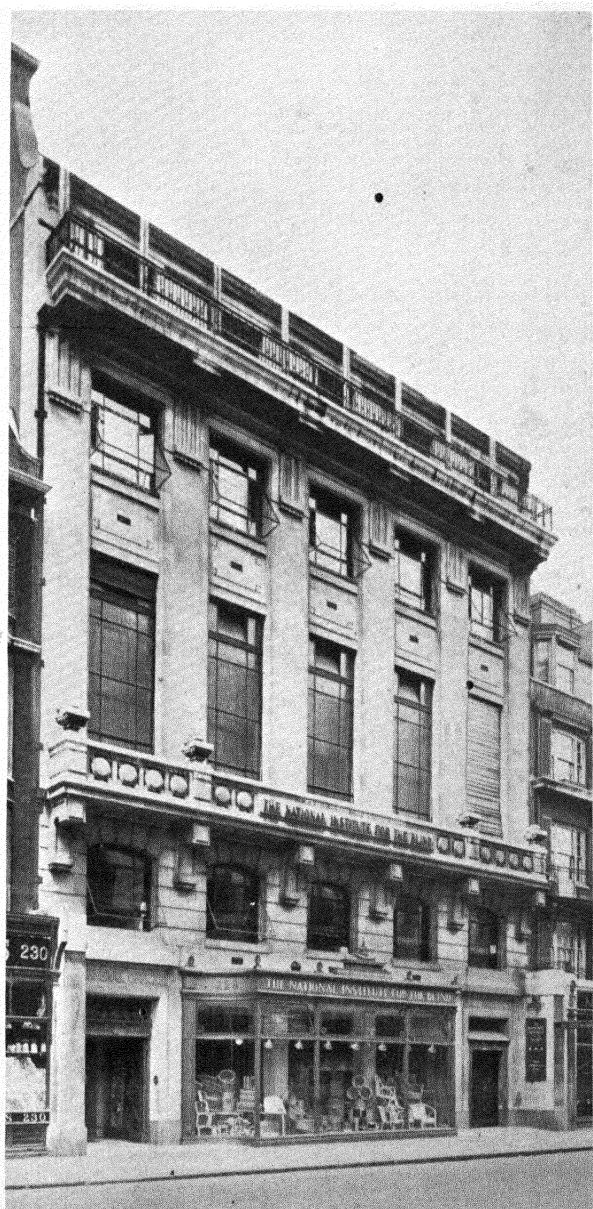
NATIONAL INSTITUTE FOR THE BLIND, HEADQUARTERS (2155)
