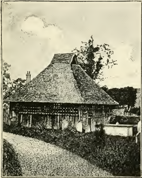
THE "BELL HOUSE" IN THE CHURCHYARD AT EAST BERGHOLT, SUFFOLK.
