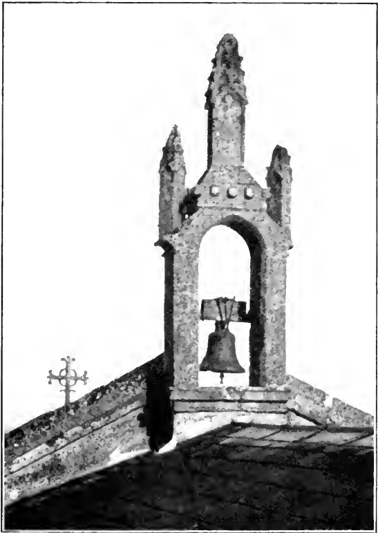
ANCIENT SANCTUS BELL (FOURTEENTH CENTURY). In its Original Cot over the Chancel Arch of Idbury Church, Oxfordshire. (See page 88).
