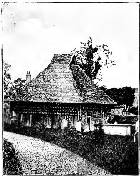
THE "BELL HOUSE" IN THE CHURCHYARD AT EAST BERGHOLT, SUFFOLK.
