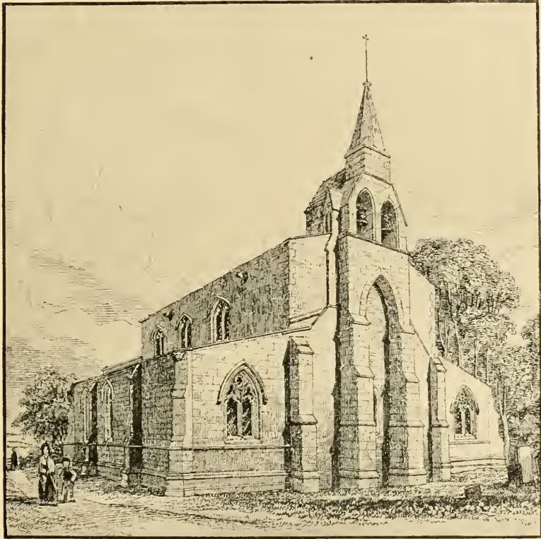
Bell-turret supported on buttresses (Burton Lazars, Leicestershire)
