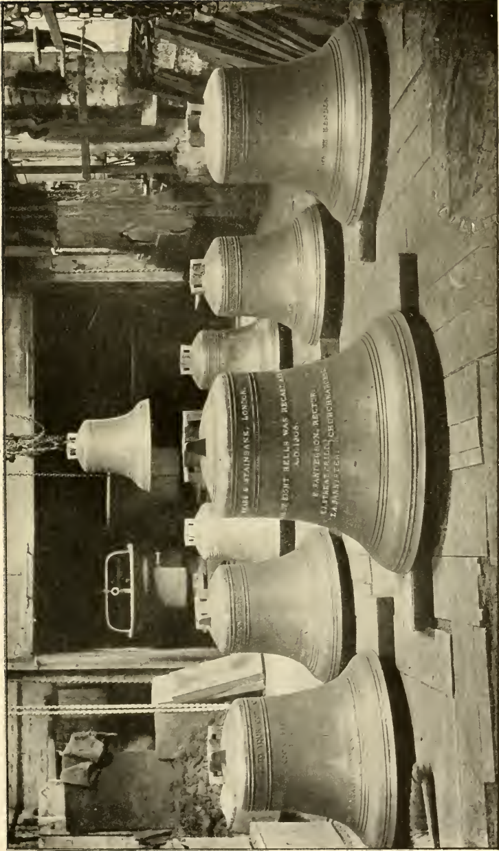
Ring of eight bells for Uckfield, Sussex, cast from the moulds already shewn
