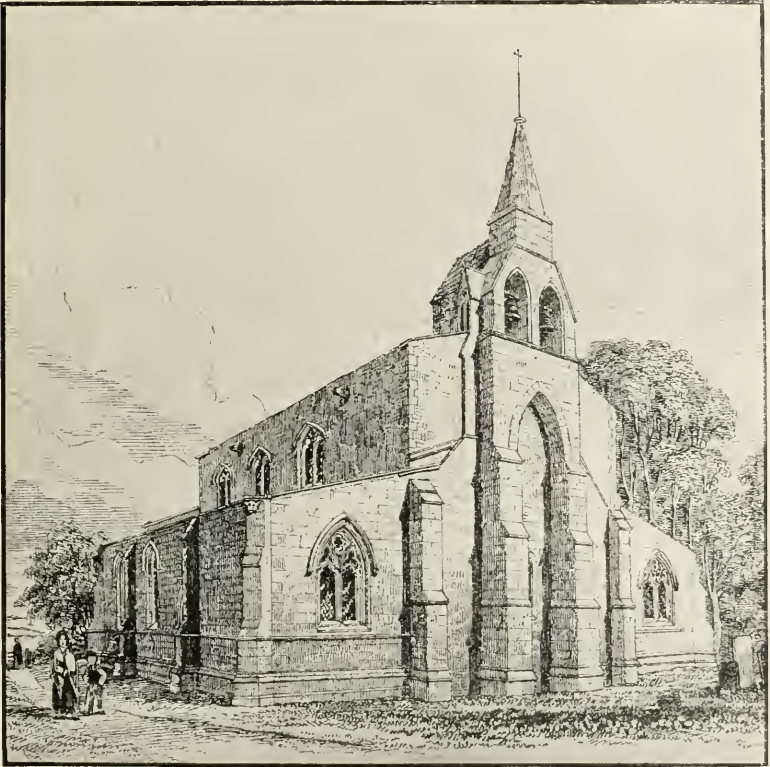
Bell-turret supported on buttresses (Burton Lazars, Leicestershire)
