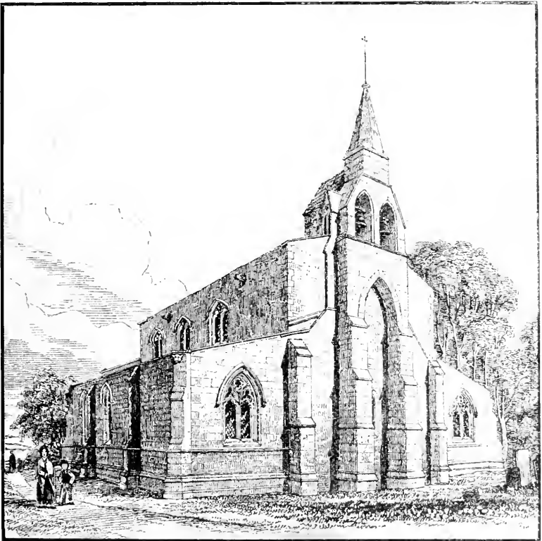
Bell-turret supported on buttresses (Burton Lazars, Leicestershire)
