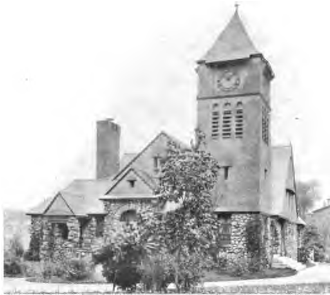
XII. EXAMPLE OF BAD STONE WORK AND AFFECTED DESIGN.
