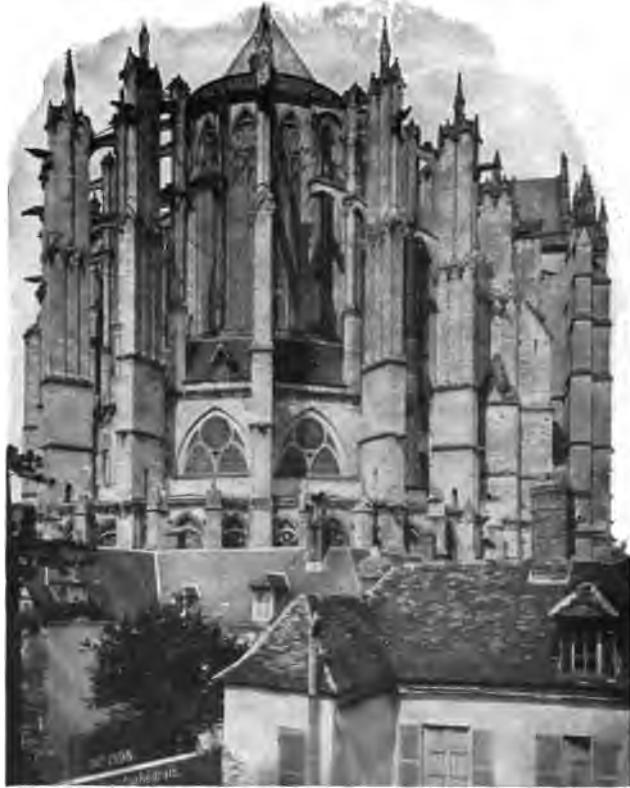
CVI. BEAUVAIS—EXTERIOR OF CHOIR.
