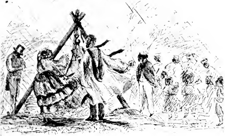
LAYING THE FOUNDATION STONE OF BIMLIPATAM CHURCH BY THE REV. J. GRIFFITHS.
