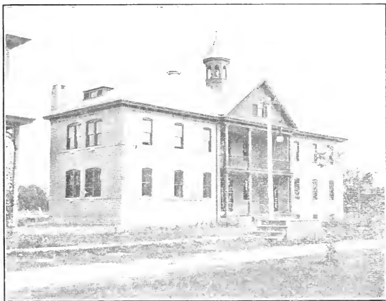
THE ASSEMBLY HALL
