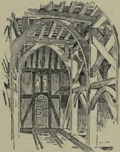
TIMBER WORK OF TOWER OF MARGARETTING CHURCH.
