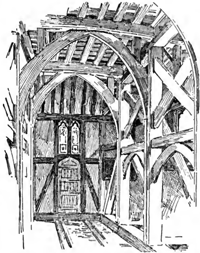
TIMBER WORK OF TOWER OF MARGARETTING CHURCH.
