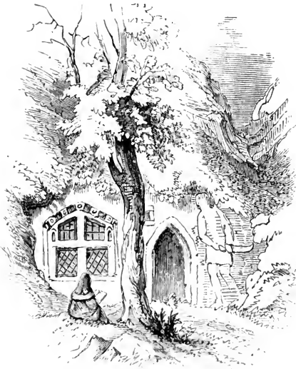
EXTERIOR VIEW OF ST. ROBERT'S CHAPEL, KNARESBOROUGH.
