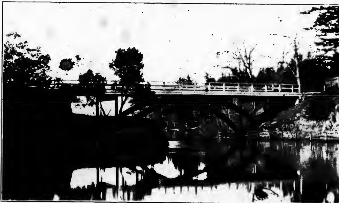
The illustration shows a Steel Arch, erected by us some years ago over Victoria Arm on Vancouver Island.
