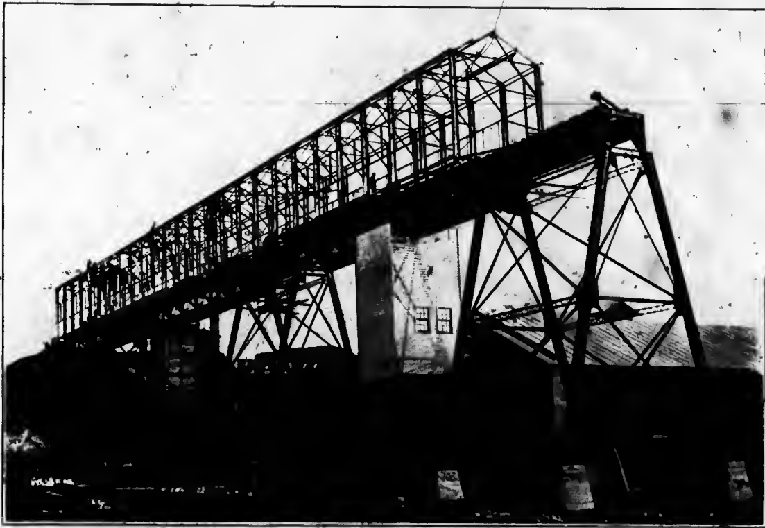
The above cut illustrates steel trestle built by us for the National Portland Cement Company, at Durham, Ontario, and was part of our general contract for steel buildings complete for this plant.
