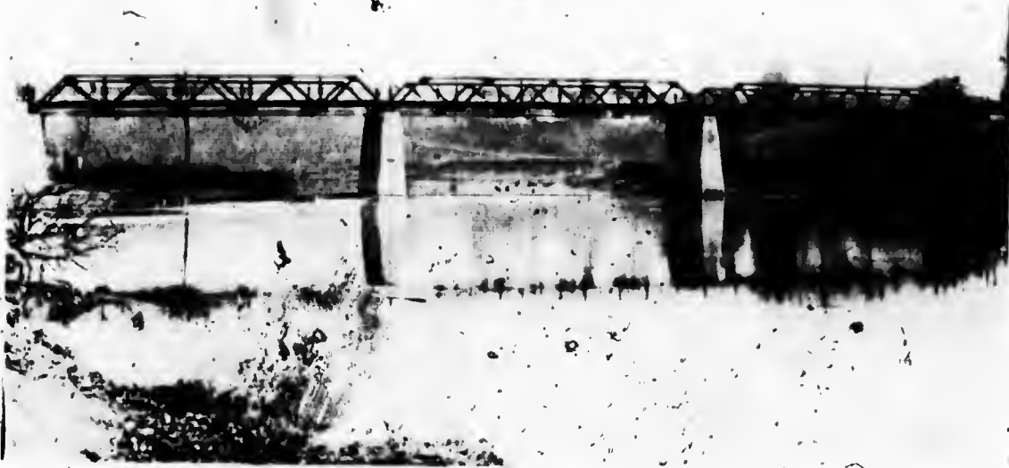
The above illustration shows three Warren Truss Steel Highway Spans, built by us near London, Ont., and known as Plover Mills Bridge.
