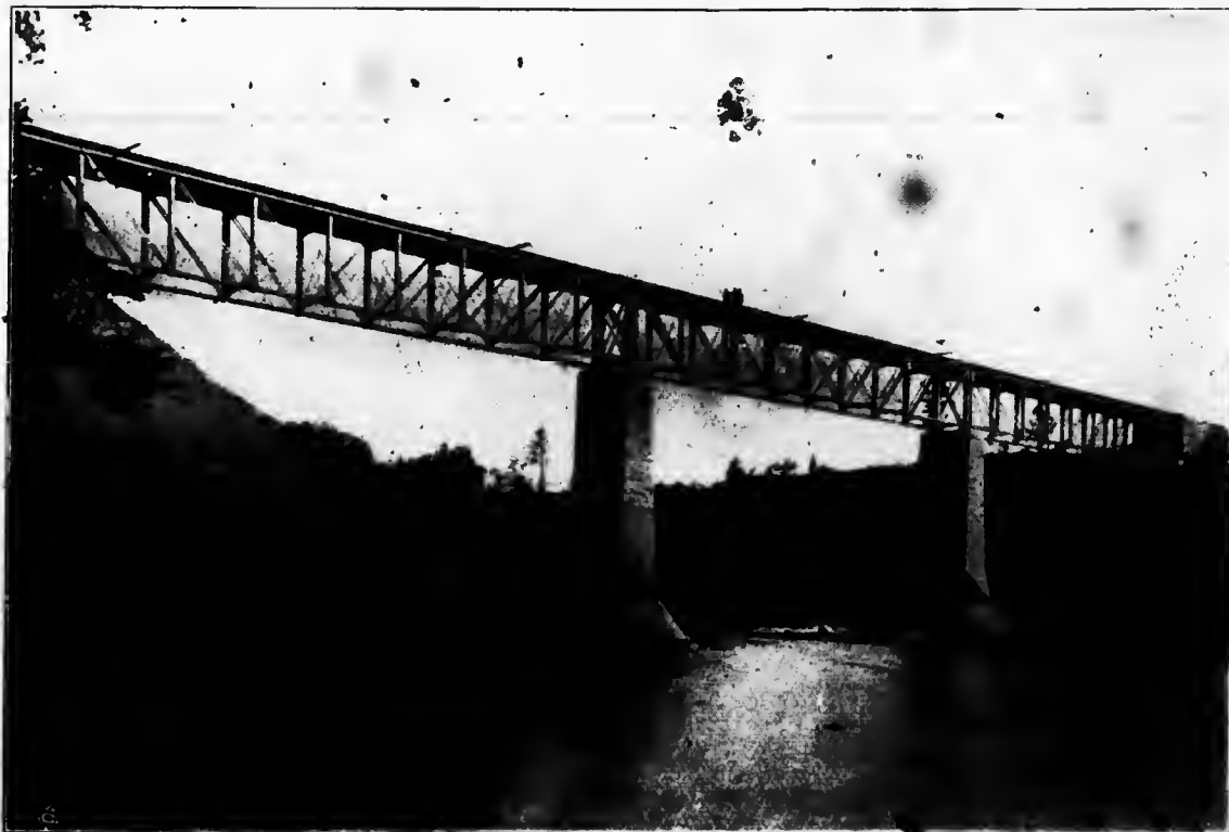
Steel Bridge over the River Humber, near Toronto, Ont., on the line of the Canadian Pacific Railway. Three spans of 157' each.
