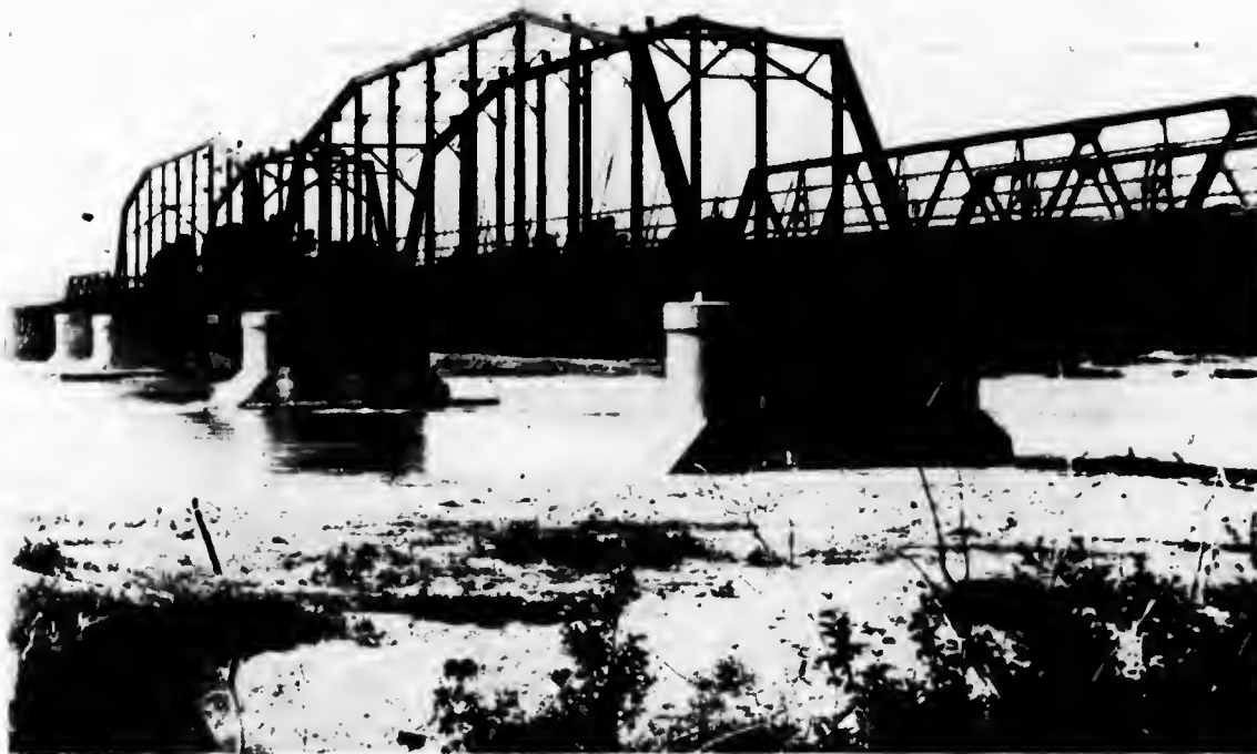
The above illustration shows a bridge built by us for the North-West Government several years ago, across the Old Man River at McLeod. It consists of two 175' Pin Connected Spans and two 80' Riveted Warren Truss Spans, all with a 16' roadway. On page No. 42 is an illustration showing the very handsome concrete piers used for Belly River, at Lethbridge, and we understand the substructure for McLeod bridge is practically the same. Page 41
