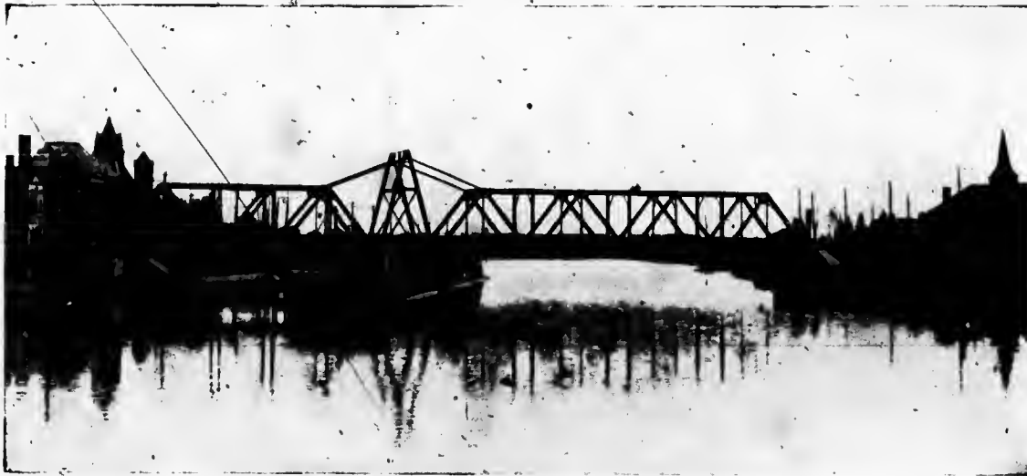
This cut illustrates a bob tail swing bridge built by us over the Welland Canal at the Town of Welland several years ago and is a very good illustration of Government practice in canal swing bridges. This is known as Alexandra Bridge.
