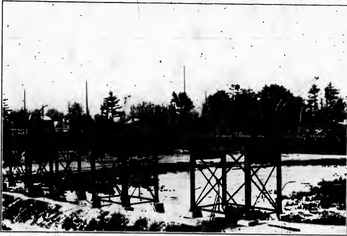
This cut illustrates a steel viaduct or trestle bridge on the line of the Hamilton Radial Railway at Oakville, Ont., and is a fine example of Electric Railway Bridge work. The structure has provision made for double track electric lines and has a sidewalk on one side.
