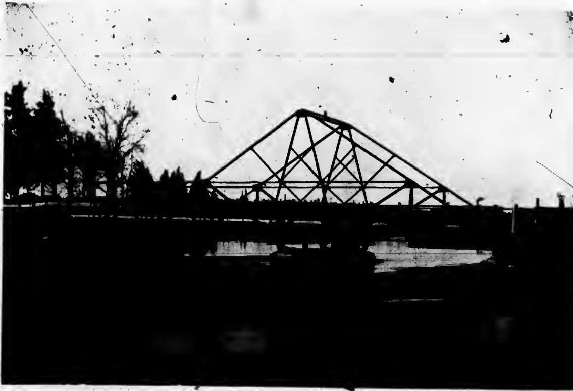
This cut illustrates a light highway swing bridge erected by us at Kemptville, some years ago, and is one of several similar spans erected in different parts of the country.
