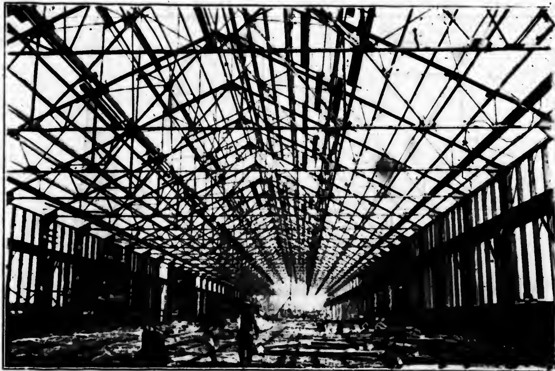
This cut illustrates the structural steel in the grey iron foundry erected by us several years ago for the International Harvester Company, of this city. So far as we know this is the longest steel building used for such purposes in Canada. The overall length of the steel is about 1000' and the width 85'. The construction consists of steel roof trusses carried on steel columns and the columns also support steel runways to handle overhead travelling cranes.
