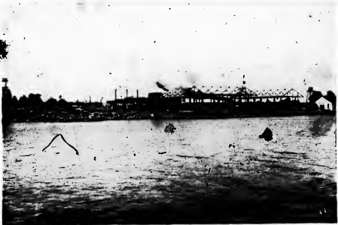
The above cut is a bird's eye view of steel buildings, erected by us, for the Belleville Portland Cement Company, at Point Ann, Ont., near Belleville. Since this cut was made we have erected several additional buildings for this plant.
