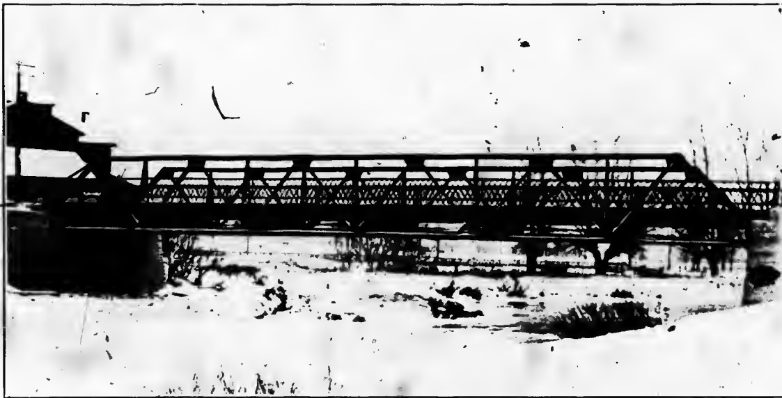
The illustration shows a 90' span erected by us in Summer of 1908, at Beachville, Ont. (and a duplicate also erected at same time for Trafalgar Township). This is a heavy span with concrete floor, lattice railings and first-class in every respect.
