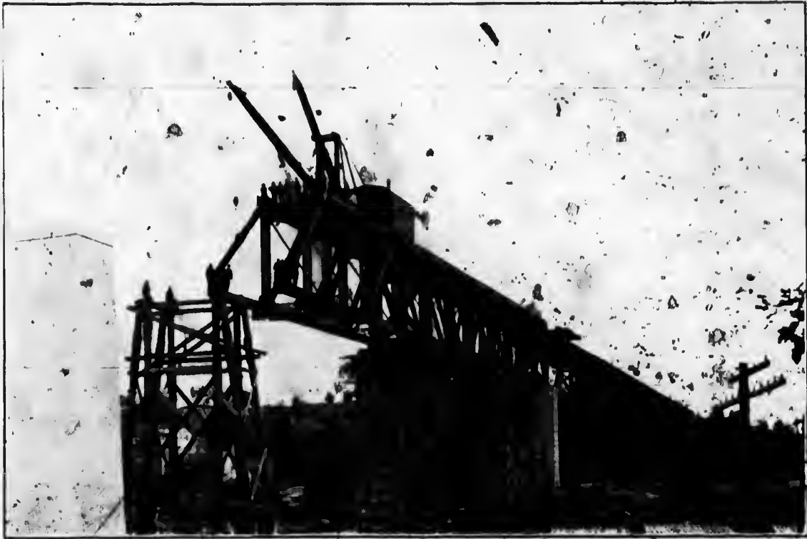
Sagin Viaduct, Parry Sound, Ont.
