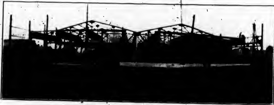
This illustration shows the steel work of our new bridge shops in the course of erection and nearly completed, and ready to receive the roofing and siding.
