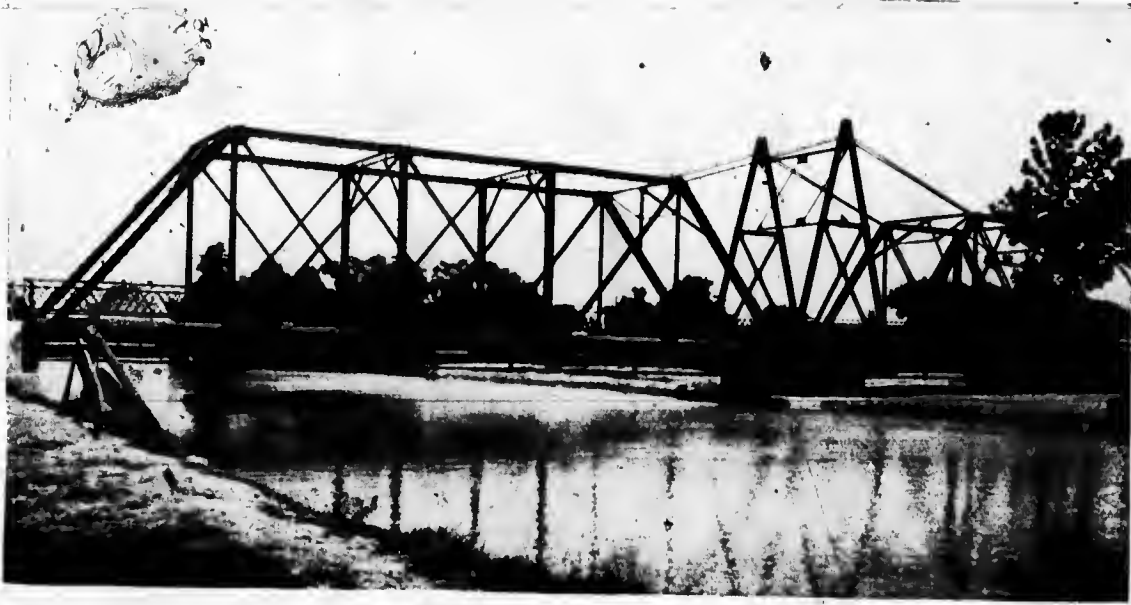
The above cut illustrates a bob tail highway swing bridge erected by us on the Welland Canal at Humberstone.
