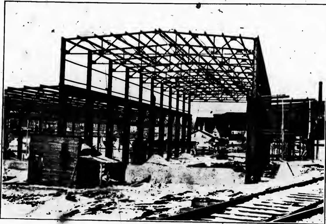
The above cut illustrates the structural steel erected by us in the new Foundry Building for the McGregor, Gourlay Company, of Galt, in 1906. This illustrates the latest type of construction used in buildings for foundry purposes. It will be noted the steel trusses are supported on steel columns and that there are steel runways to support heavy travelling crane.
