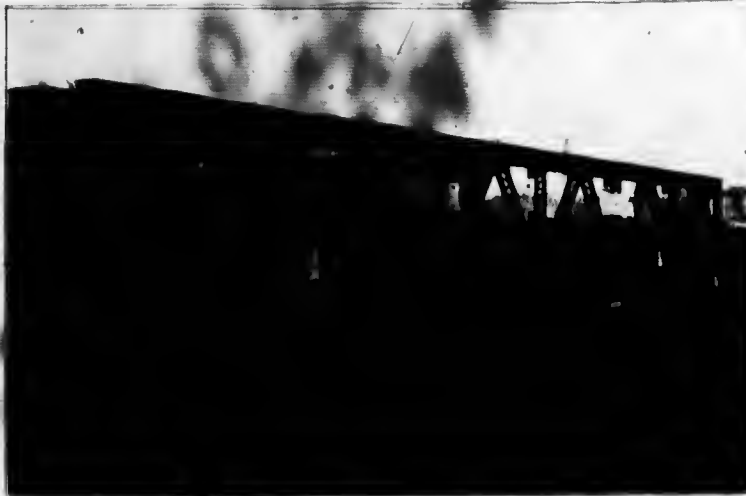
The above illustration shows a single lattice girder 130' span riveted up complete and shipped to its destination where it was connected and riveted up with another girder and placed in position complete.
