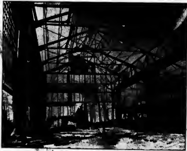
The above cut shows an interior view of steel building for Open Hearth Plant of the Hamilton Steel & Iron Company. Since the erection of this building, several additions have been added at each end.
