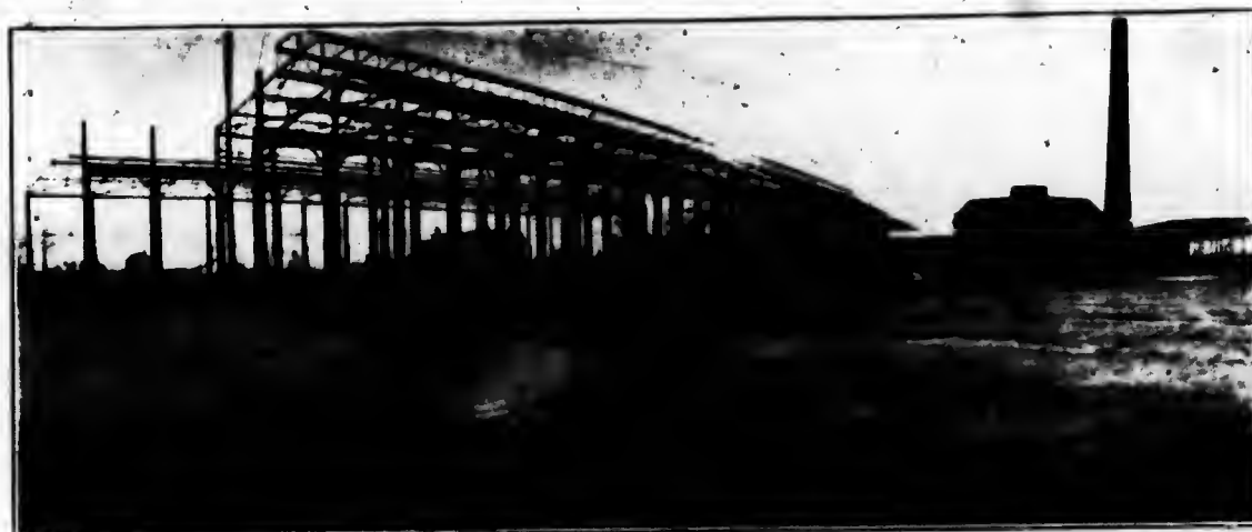
The above cut illustrates structural steel of Machine Shop for the Canada Foundry Company, at Toronto, being a part of the contract we had for several other buildings in connection with this plant.
