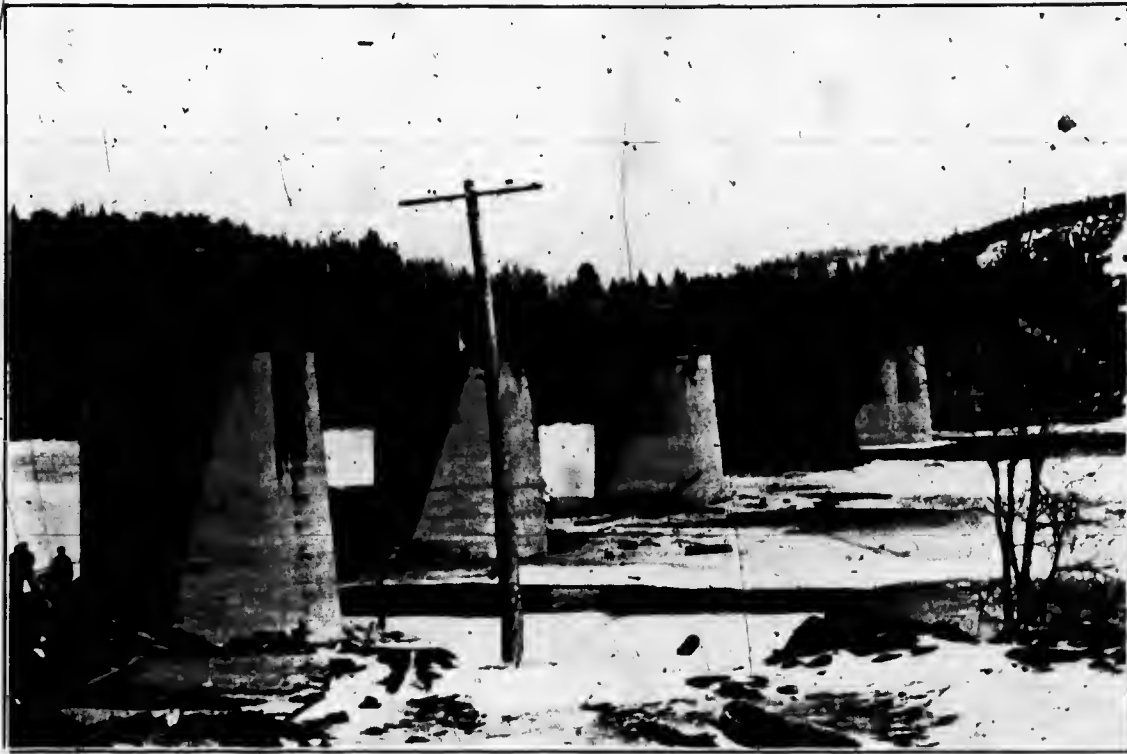
The above illustration represents a bridge on the line of the Canadian Pacific Railway at Aroostook Junction, N. B. This was a case in which our contract covered the removal of four through plate girder steel spans and replacing three of them with deck plate girder spans and the removal of the fourth to the far end of the bridge, and also putting in several additional girders.
