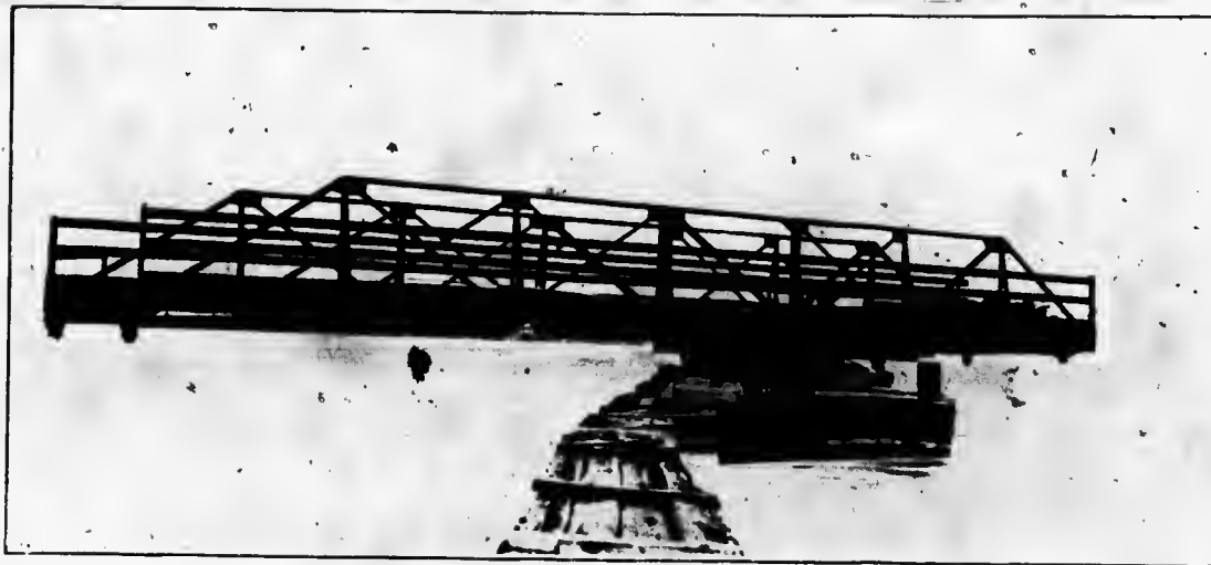
This cut illustrates a light highway swing bridge erected by us, several years ago, at Chemong, being part of the floating bridge at that point, and is very similar in design to that shown on page No. 49, with the exception that overhead bracing is omitted. This makes a very good type of light highway swing.
