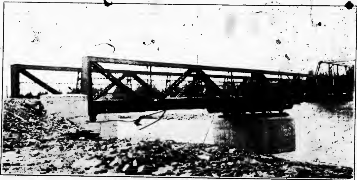
The above cut illustrates the Dominion Government Standard Highway Swing Bridges used at various points on the Trent - Valley Canal. The bridge illustrated was recently completed by us at Glen Miller, on the Trenton section of this canal, and is one of eleven similar spans erected at different points on the Simcoe-Balsam Lake Division and Holland River and Trenton sections of this canal.
