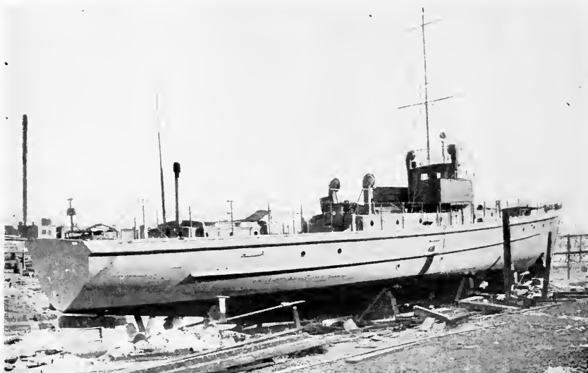
A completed Chaser waiting her turn at the launching ways.
