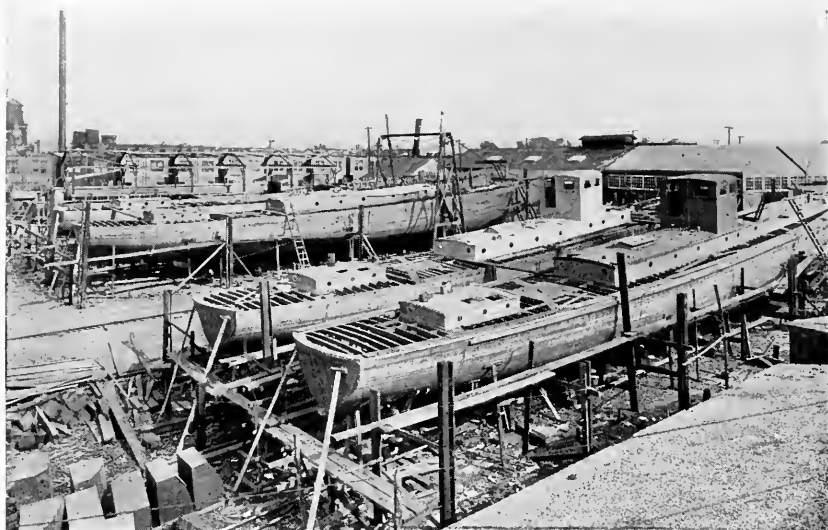
Motors installed and ready for the decks.
