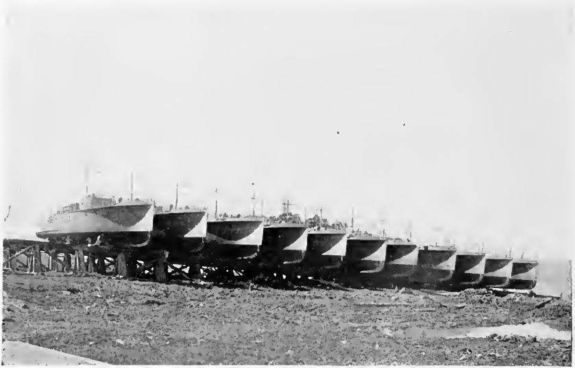
A group of M. L.'s on the ways ready for launching.
