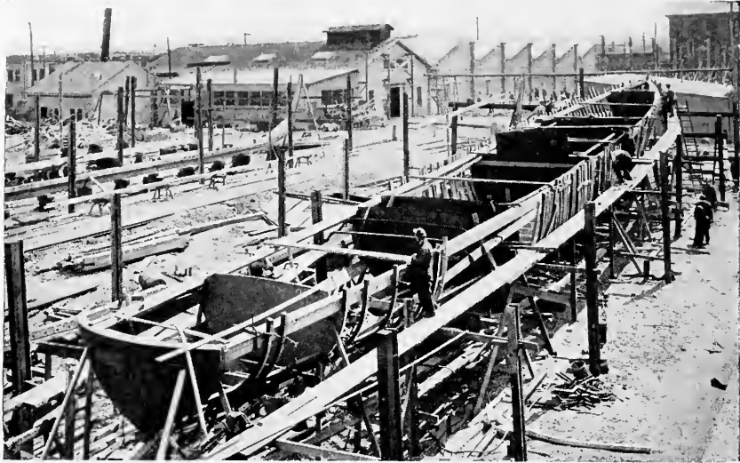
The steel bulkheads were set up on the keelson and used as molds.
