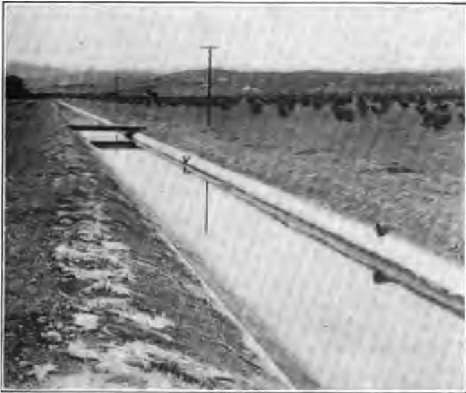
FIG. 55. — Canal lined with cement. Transformation of desert hills into orange groves.
