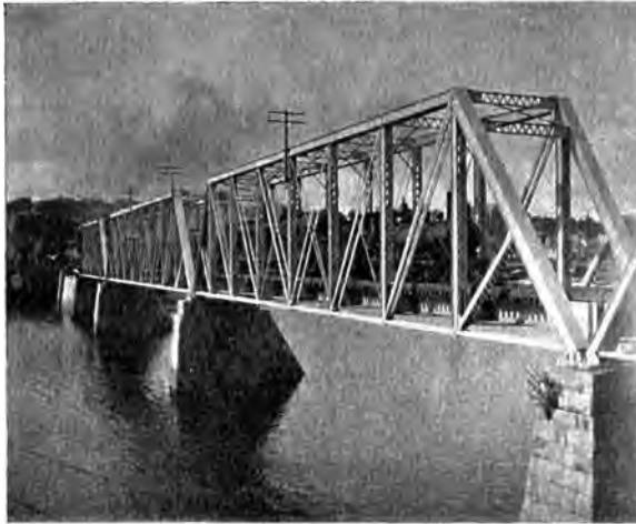
M. C. R. BRIDGE OVER THE PENOBSCOT.
