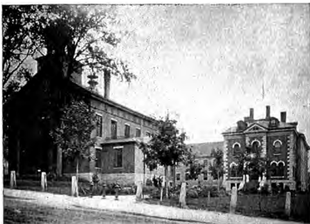
COURT HOUSE AND JAIL.
