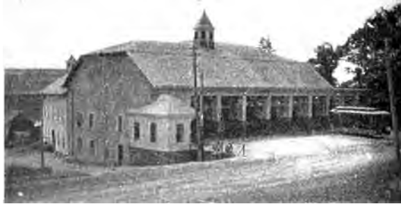
PUBLIC WORKS COMPANY'S CAR HOUSE.
