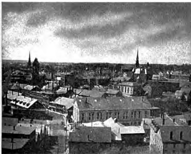
THE WEST SIDE, FROM AN EAST SIDE VANTAGE GROUND.
