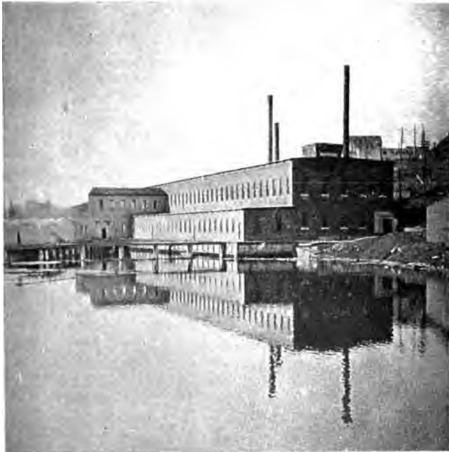
PUBLIC WORKS COMPANY'S POWER STATION AT VEAZIE.
