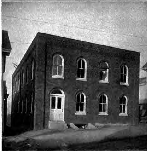
SUB-STATION, PARK STREET.
