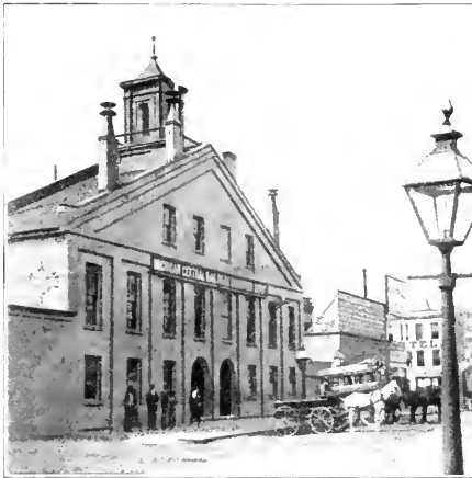
MICHIGAN CENTRAL DEPOT, 1853-53
