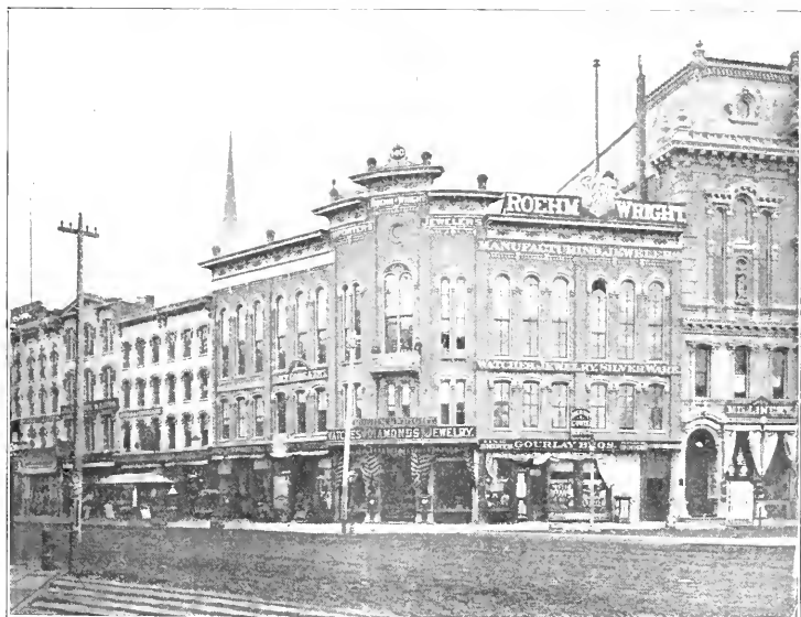
NORTHEAST CORNER WOODWARD AND CAMPUS MARTIUS ABOUT 1881 Corner building still standing
