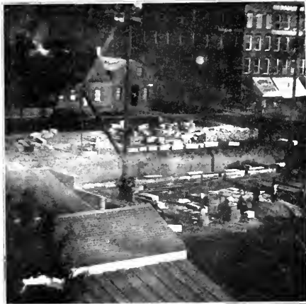
EXCAVATION FOR OLD POST OFFICE ON GRISWOLD AND LARNED
