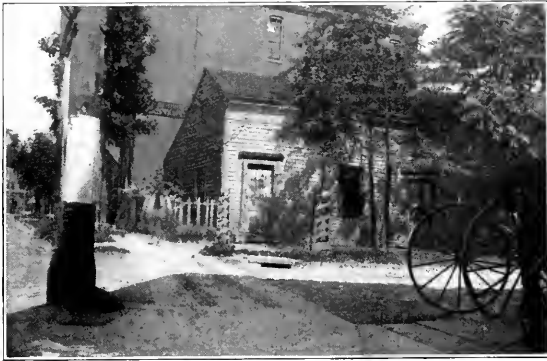
SOUTHEAST CORNER FARMER AND JOHN R STREETS House built about 1811
