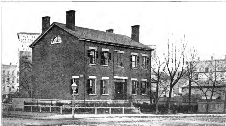
OLD ABBOTT HOMESTEAD, SOUTHEAST CORNER OF GRISWOLD AND FORT Built in 1835; torn down in 1881. Now site of the Hammond Building
