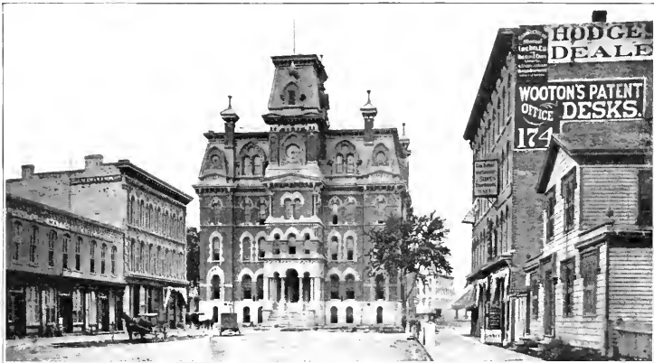
OLD DETROIT HIGH SCHOOL AT HEAD OF GRISWOLD STREET, WHERE CAPITOL PARK IS NOW LOCATED Formerly the State Capitol Building but remodeled for school purposes
