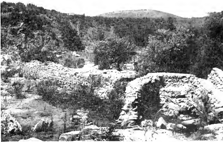
RUINS OF THE OLD MISSION DAM Built by the Franciscan Fathers.
