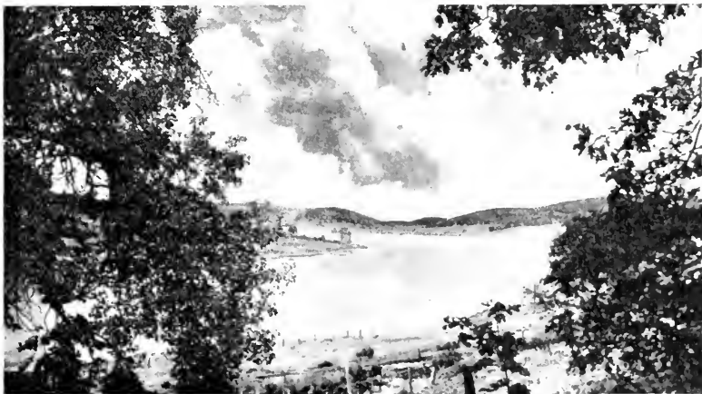
CUYAMACA LAKE, PART OF CUYAMACA WATER SYSTEM
