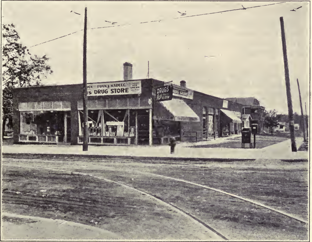
A set-back of a new building on a future arterial street, Minneapolis
