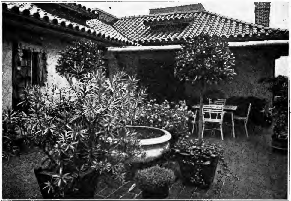
New York Roof Garden and Penthouse
