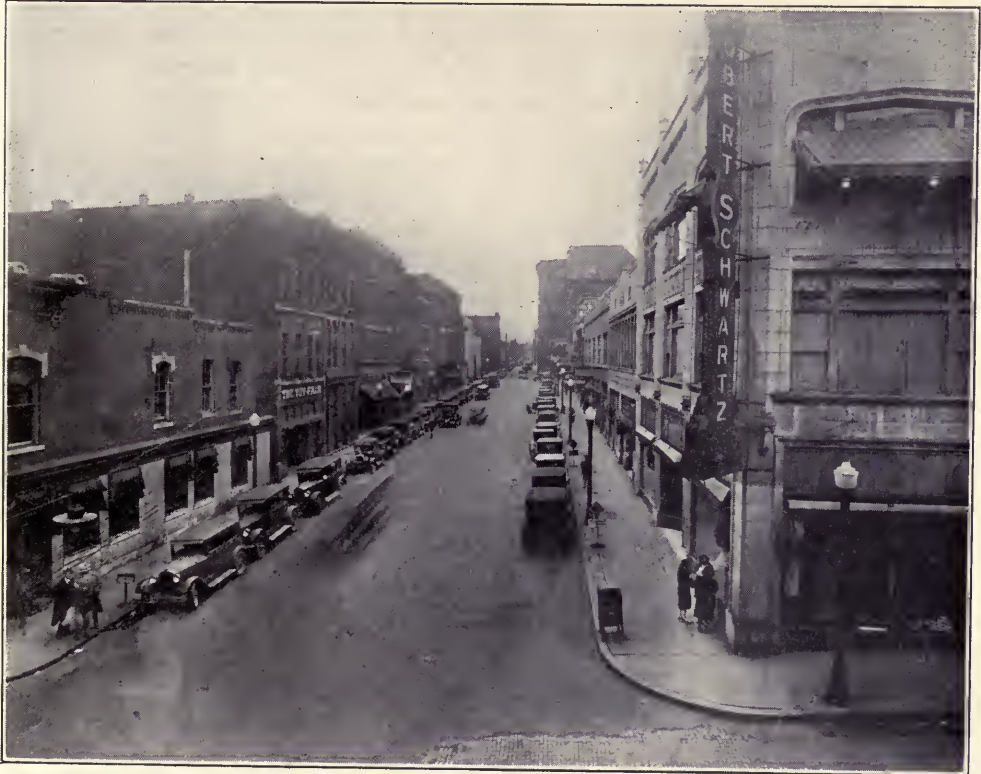
Before and After, Cherry Street Widening, Chattanooga
