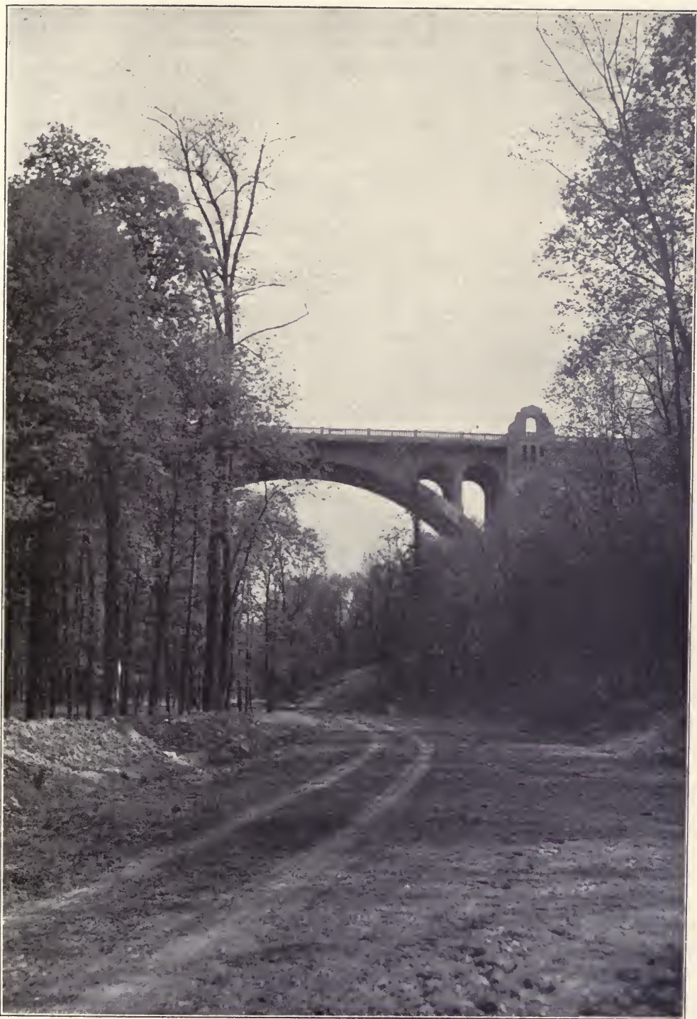
HILLIARD ROAD BRIDGE OVER ROCKY RIVER PARK Separation of park and highway traffic in the Cleveland Metropolitan Park System
