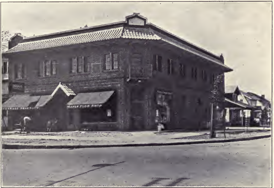
Deleterious Effects of Store in Residential Neighborhood Minimized by Adequate Setback
