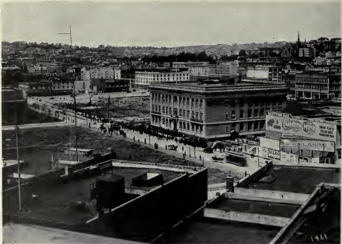
SAN FRANCISCO.—The Civic Center Site Before It Was Cleared.
