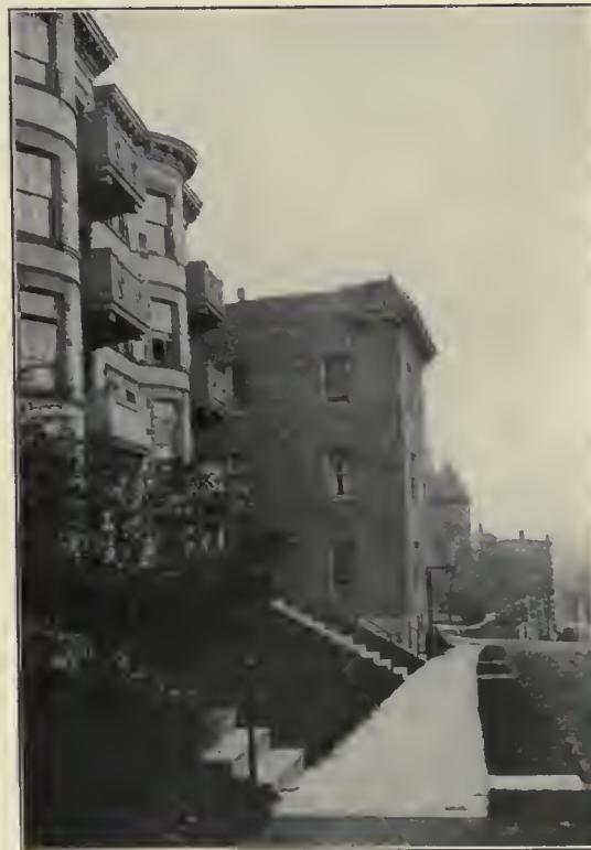
BROOKLINE.—An Apartment House Projected into the Accepted Set-back Area.
