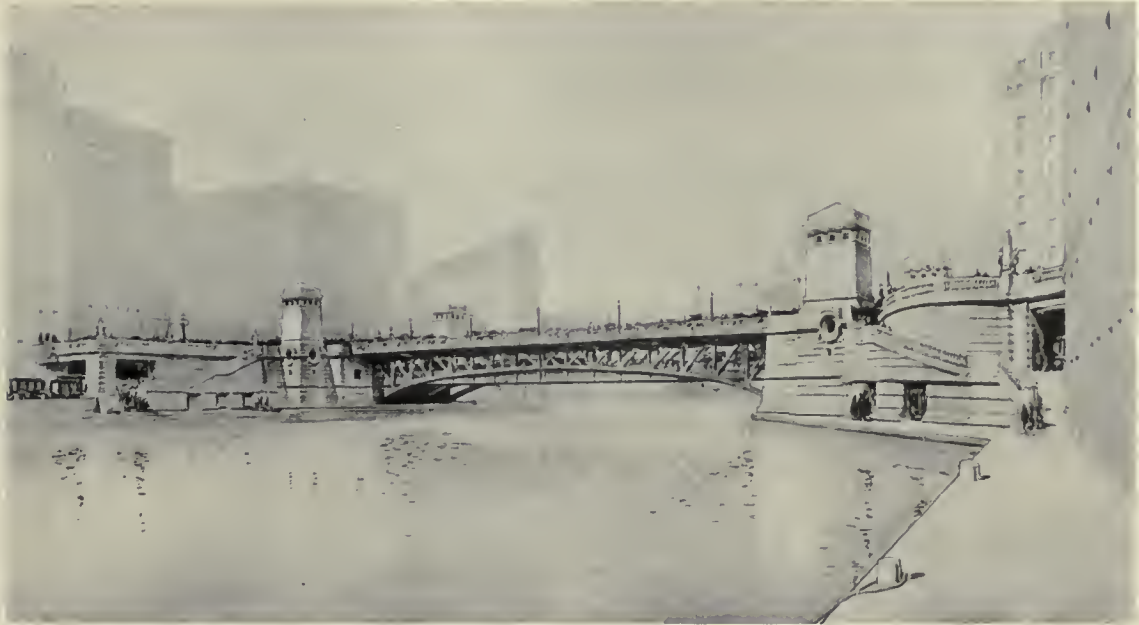
CHICAGO.—Two-level Bascule Bridge in Line with Michigan Avenue and Across the Chicago River.
