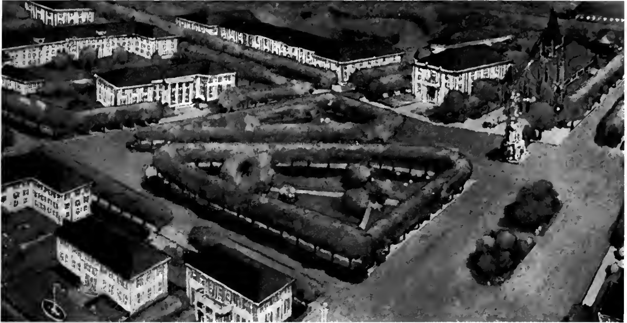
BRIDGEPORT.—Bird's-Eye View of Proposed Civic Group, Including a Site for the City Hall, Post Office, Fire Headquarters, Library, and Other Buildings.
