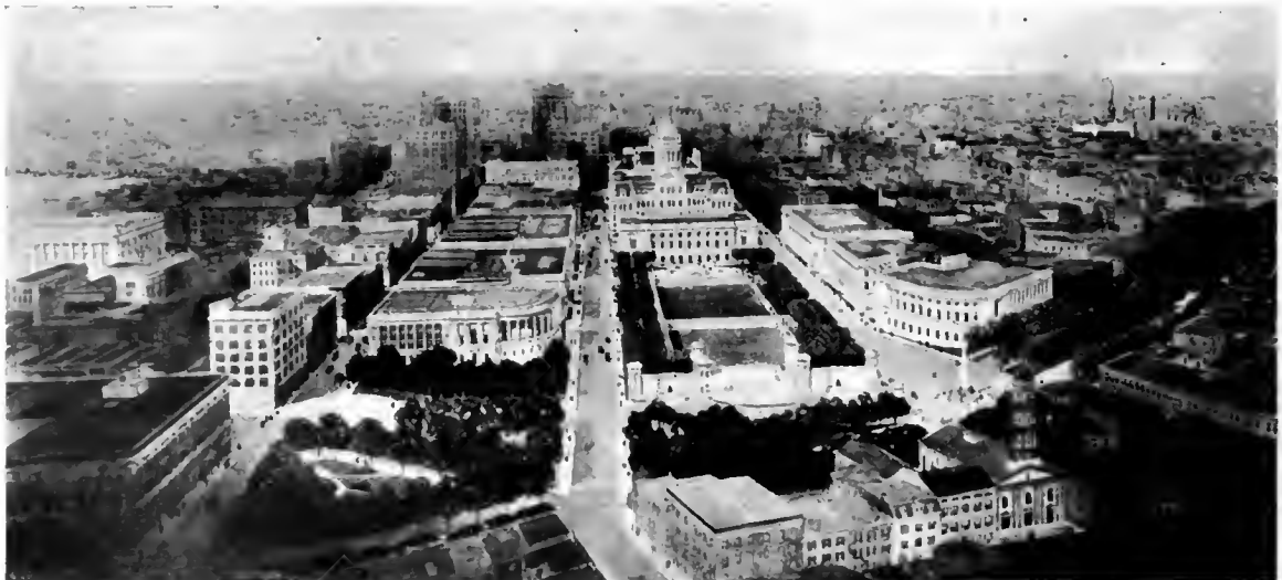
BALTIMORE.—The Civic Center Now Being Constructed with Appropriations Made Annually by the City.
