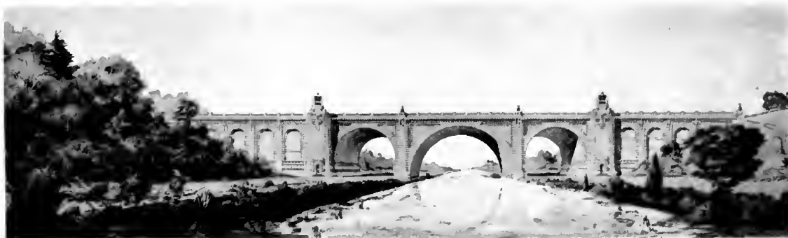
PHILADELPHIA.—New Pennypack Creek Park Bridge in Lincoln Highway.
