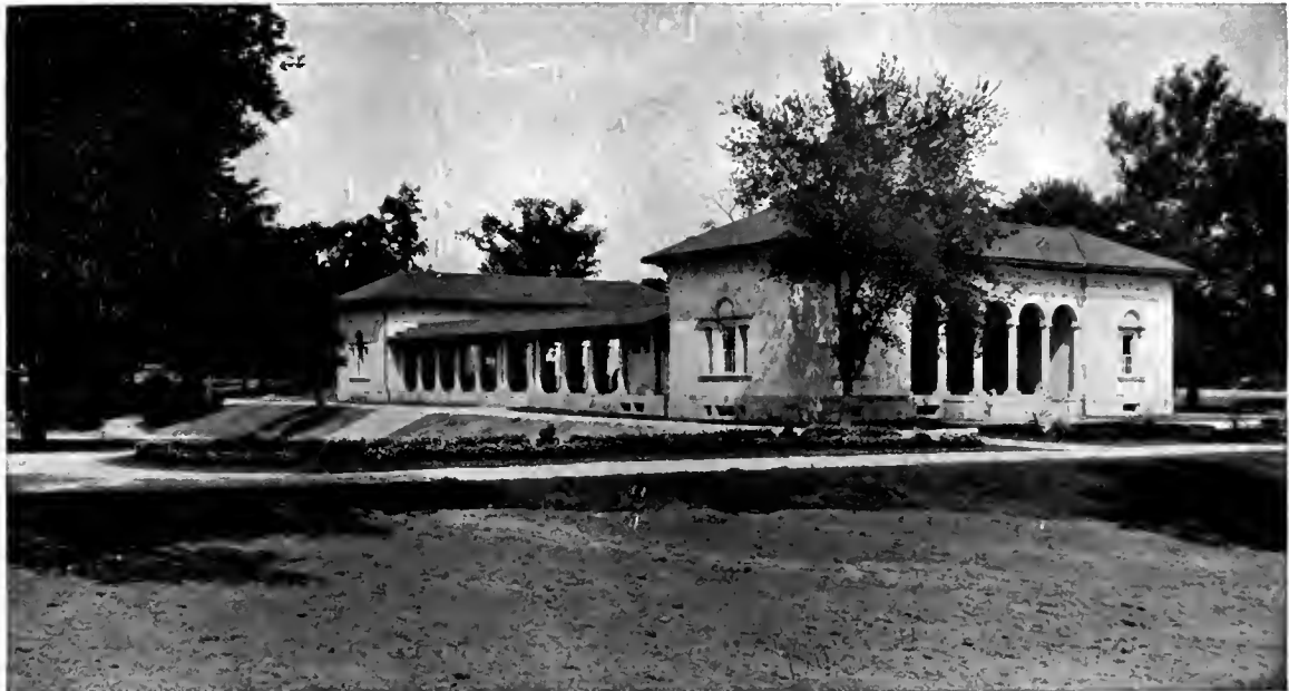
KANSAS CITY.—Bathhouse in the Grove; the Most Complete Combined Park and Playground in the City. Area of Park, 11 Acres; Entire Cost, $283,000.
