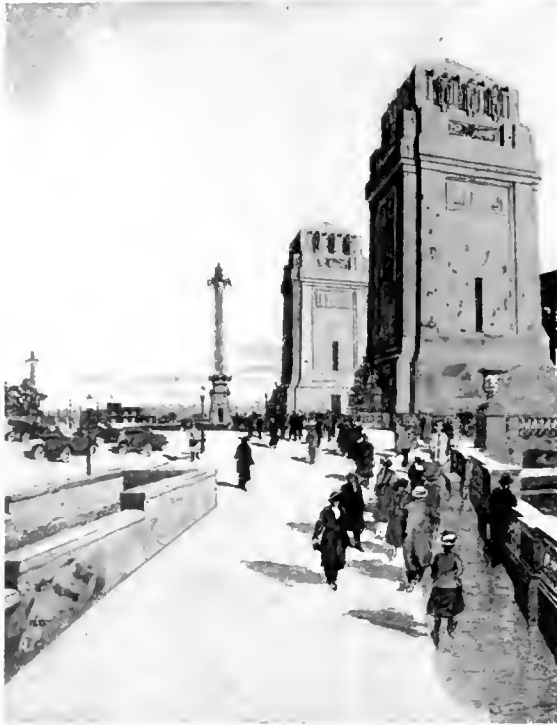
CLEVELAND.—Bridge Pylons and Plaza to High-Level Bridge.
