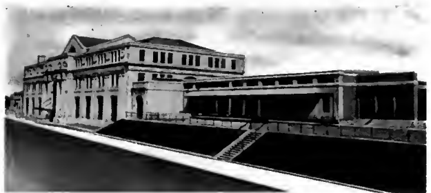
MACON.—New Passenger Terminal, with Well-Ordered Approaches and Attractive Architectural Treatment.
