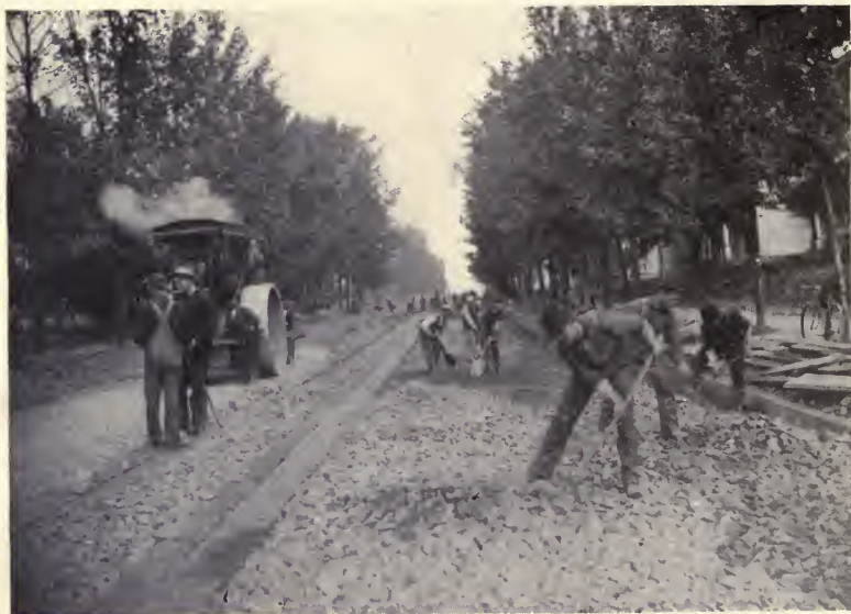
NORTH JAMES STREET, ROME, N. Y. Laying bituminous foundation or base.
