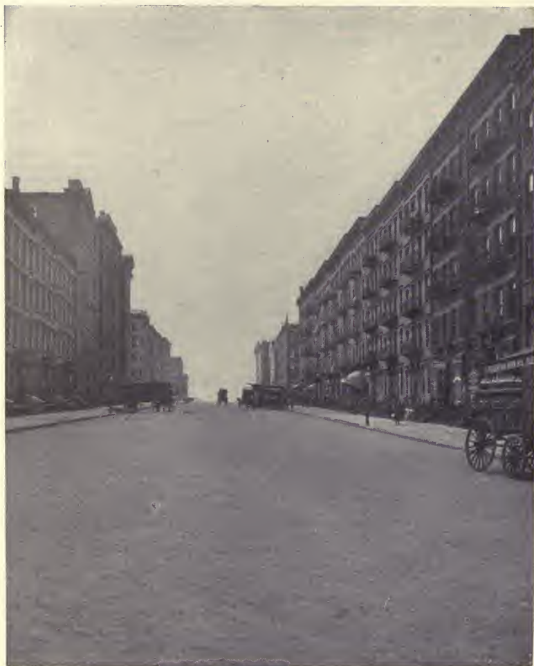
BLOCK ASPHALT PAVEMENT, NINETY-SIXTH ST., NEW YORK, 1900. Looking west from Third avenue to Park avenue. Paved in 1900.
