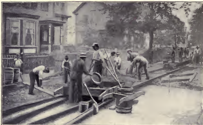
Mixing and placing concrete base.
