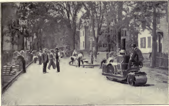
Rolling with two and one-half ton roller.
