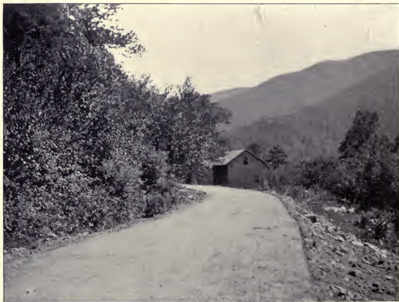
Sandstone or "bluestone" road, built in Ulster county, N. Y., in 1900.
