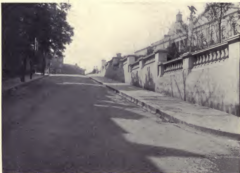
BOWDOIN STREET, BOSTON, MASS. Bitulithic pavement laid on 13 per cent grade in 1902.
