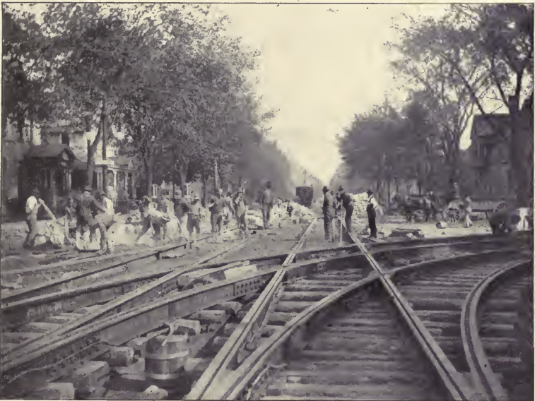
TRACK AND PAVEMENT CONSTRUCTION, ROCHESTER, N. Y., 1900.
