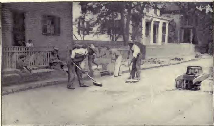
Spreading Portland cement grout filler.
