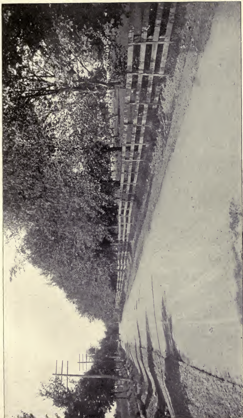
VANDENBURGH AVENUE, TROY, N. Y., 1901. Surface of trap on base of four inches of limestone.
