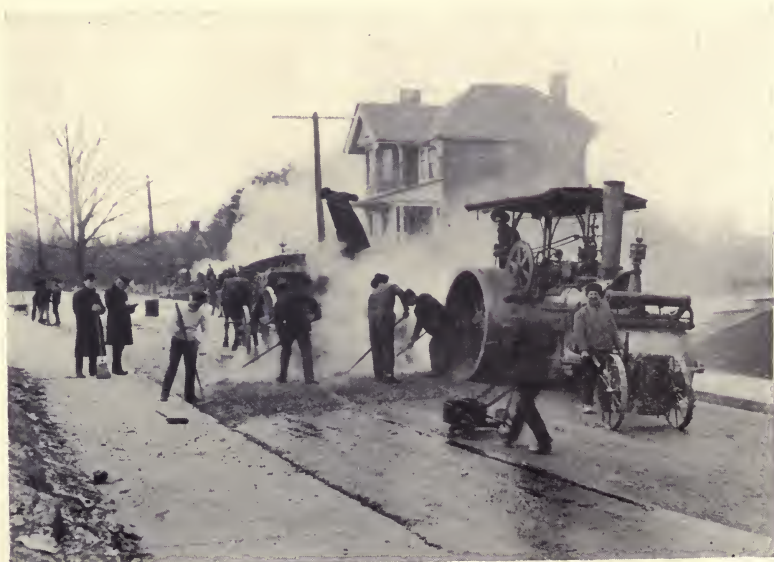
WOODLAWN AVENUE, TORONTO, ONT. Laying Bitulithic surface.
