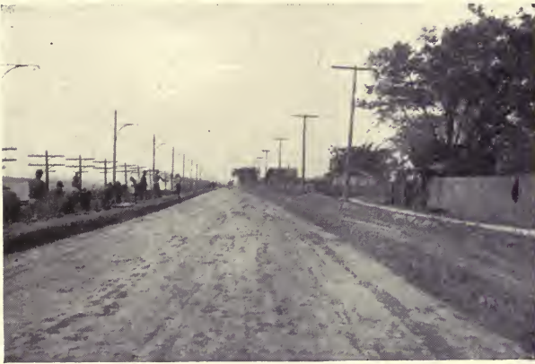
Finishing subgrade.
