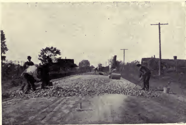
Spreading and binding foundation stone.
