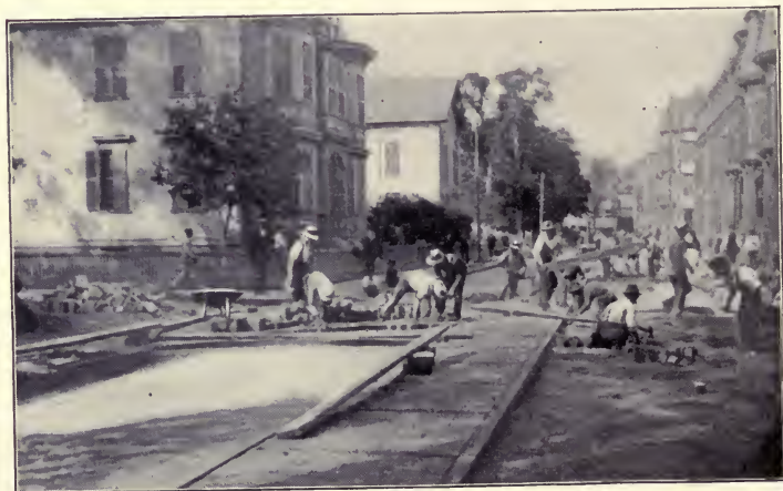
Placing brick on sand cushion.
