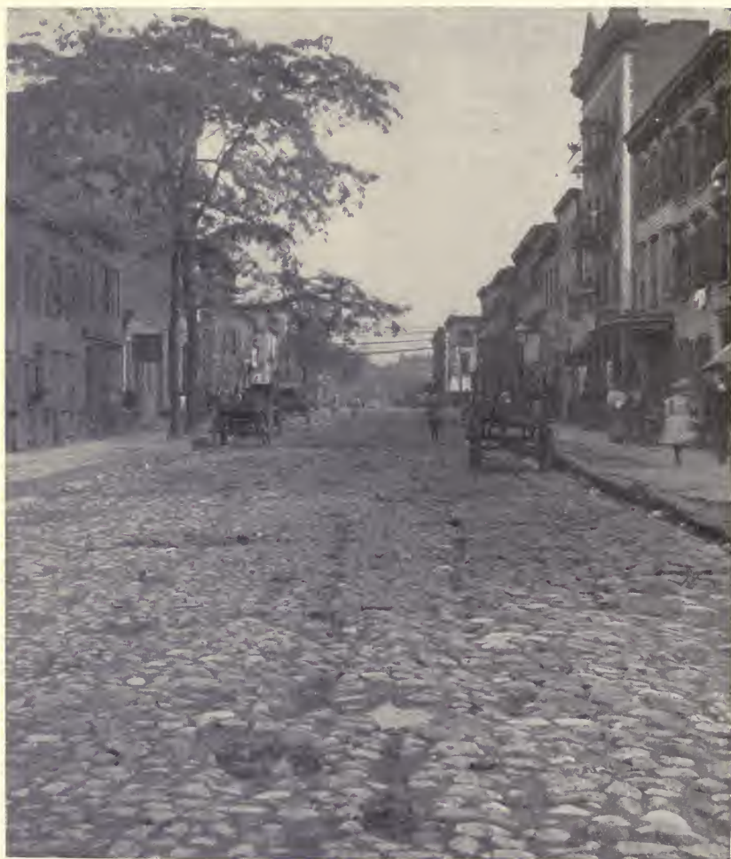
CARROLL STREET, BROOKLYN, NEW YORK, 1900. Before covering cobble pavement with sheet-asphalt in 1900.
