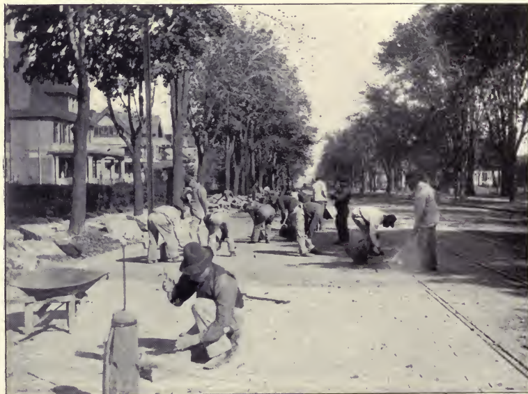
Filling joints with coarse sand and hot paving cement.
