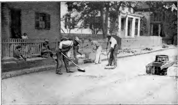
Spreading Portland cement grout filler.
