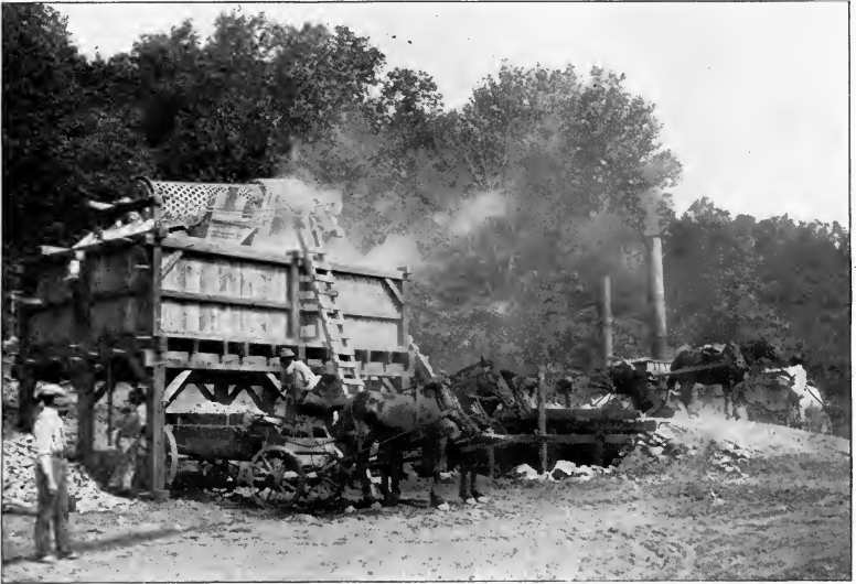
Tailings larger than 3 inches to return to crusher.
