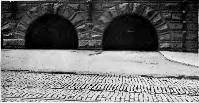
Brick at entrance to Union Station, laid in 1893. (Stone-block pavement in foreground).
