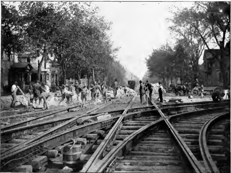
TRACK AND PAVEMENT CONSTRUCTION, ROCHESTER, N. Y., 1900.
