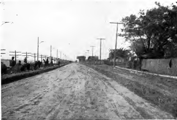
Finishing subgrade.
