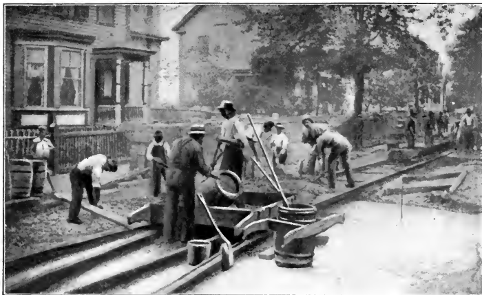
Mixing and placing concrete base.
