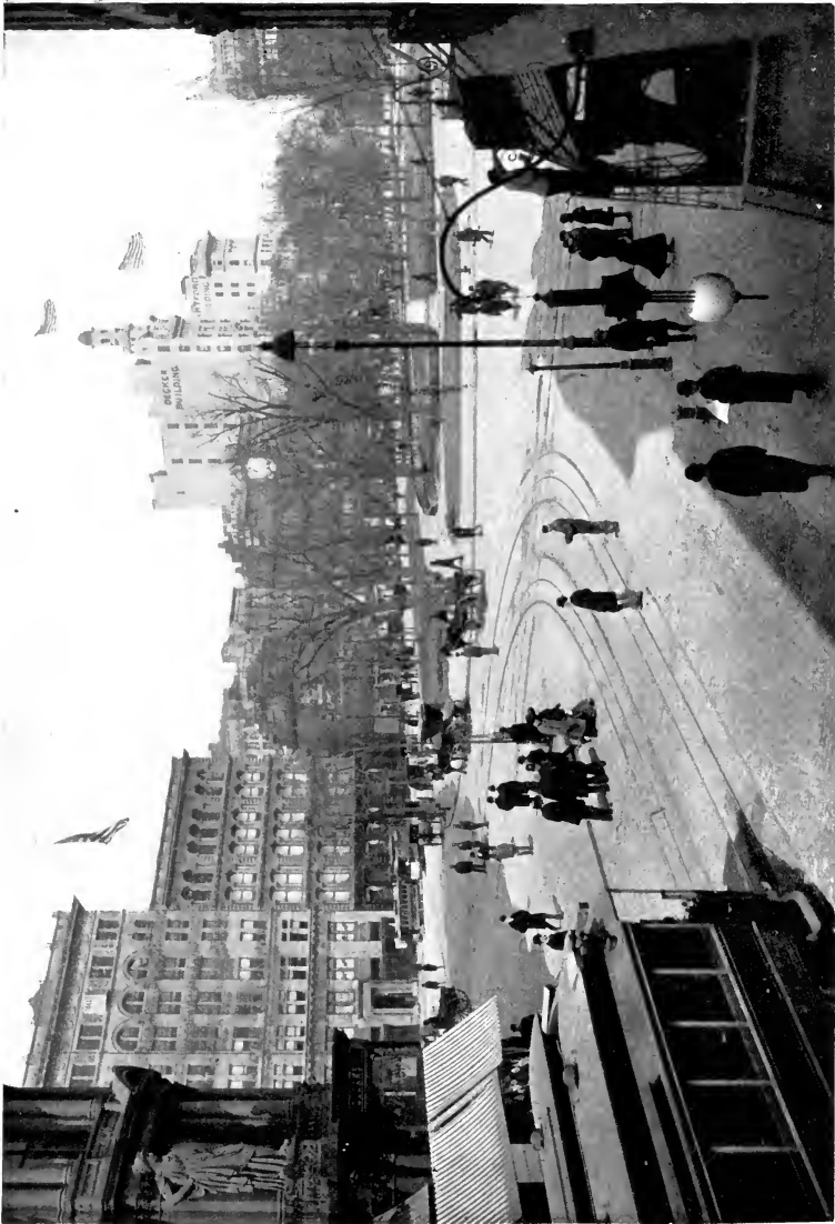
UNION SQUARE, NEW YORK, 1900. Looking up Broadway at Fourteenth Street : after paving with sheet-asphalt in 1900 : Trinidad Lake wearing surface, 2 inches : Bermudez Lake binder-coat, 1 inch.
