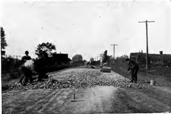
Spreading and binding foundation stone.
