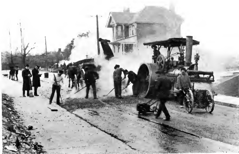
WOODLAWN AVENUE, TORONTO, ONT. Laying Bitulithic surface.
