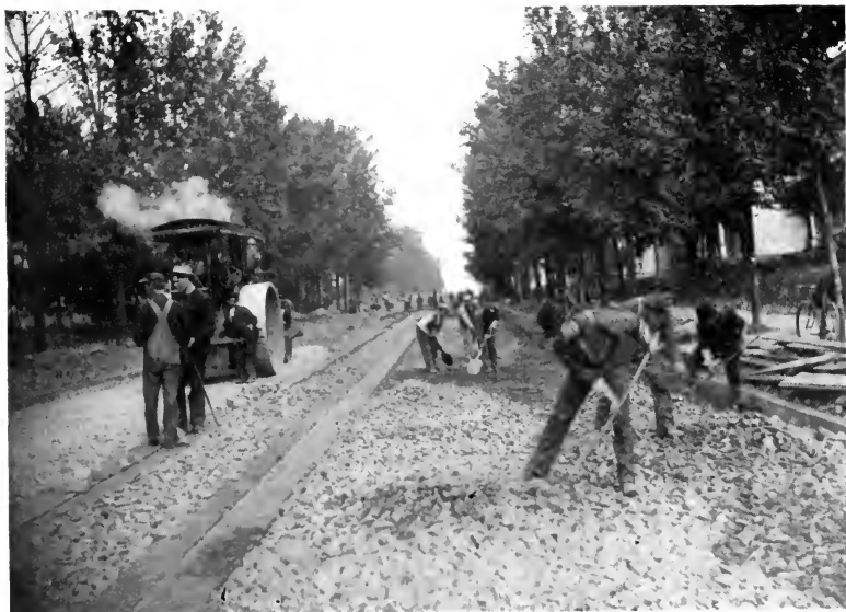
NORTH JAMES STREET, ROME, N. Y. Laying bituminous foundation or base.
