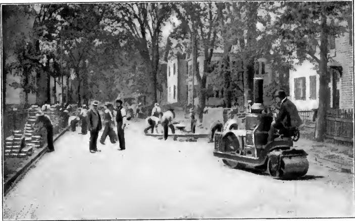
Rolling with two and one-half ton roller.
