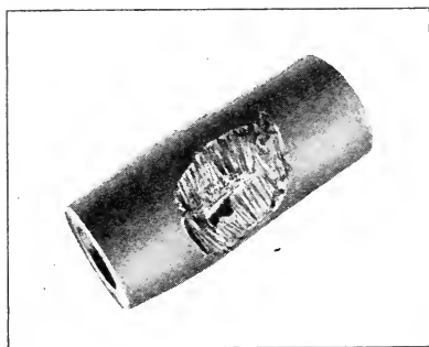
FIG. 85. Lead pipe gnawed by rats
