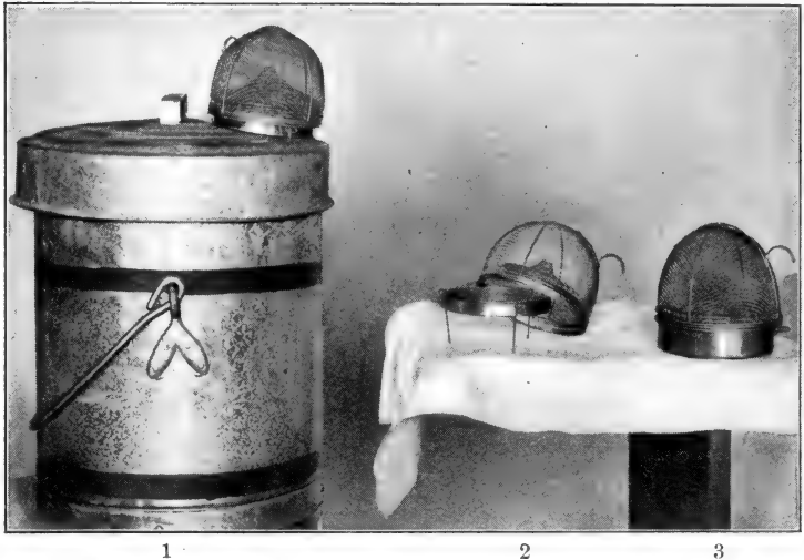
FIG. 59. Outdoor fly exterminator as adopted for manufacture
