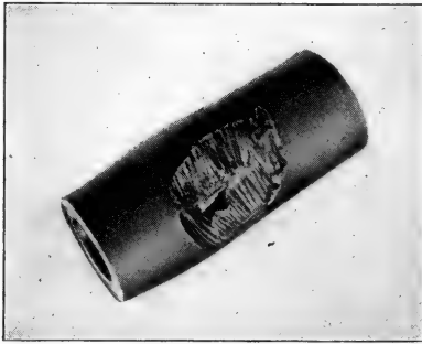
FIG. 85. Lead pipe gnawed by rats
