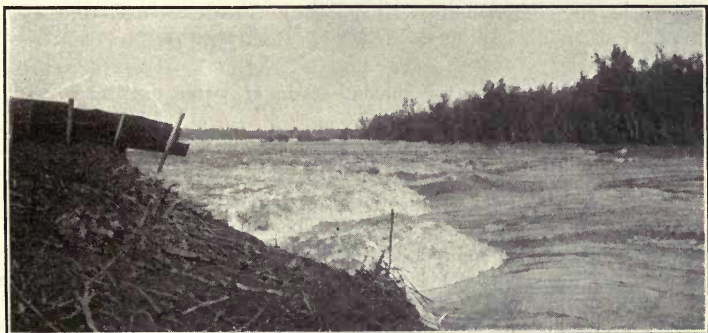
A break in the levee on the lower Mississippi.
