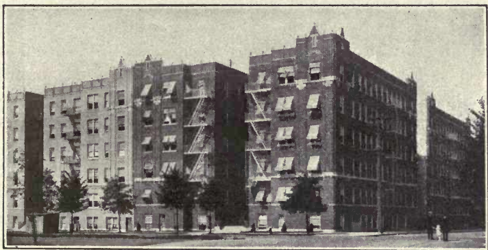
Modern apartments: fire laws respected.
