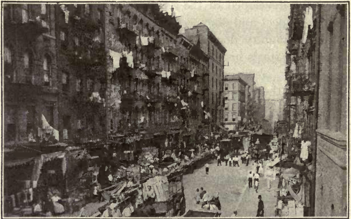
Many old tenement buildings lack proper fire escapes and often where they exist they are loaded with rubbish contrary to city regulations.
