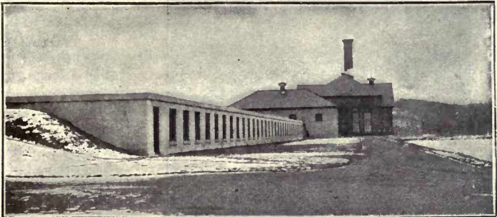
A modern filtration plant.
