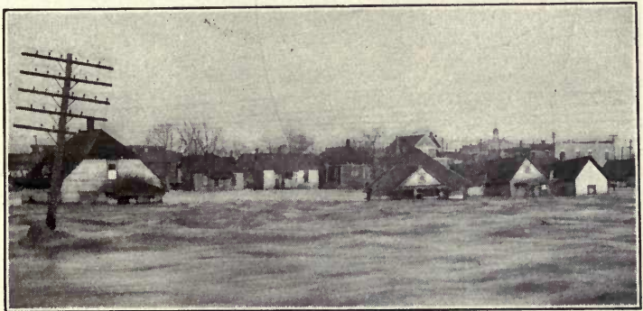
This photo was taken in Macksville, Indiana, on March 28, 1913.
