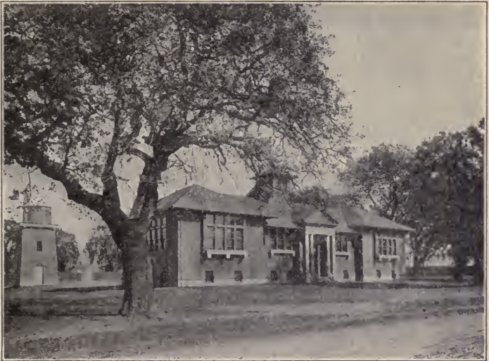
TYPICAL RURAL SCHOOL BUILDING, SONOMA COUNTY, CAL.
