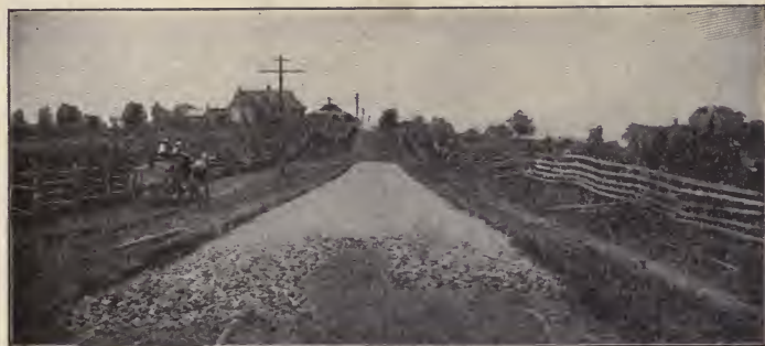
2. Laying the foundation course.
