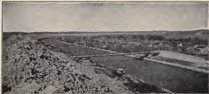
3. The Chicago Drainage Canal.
