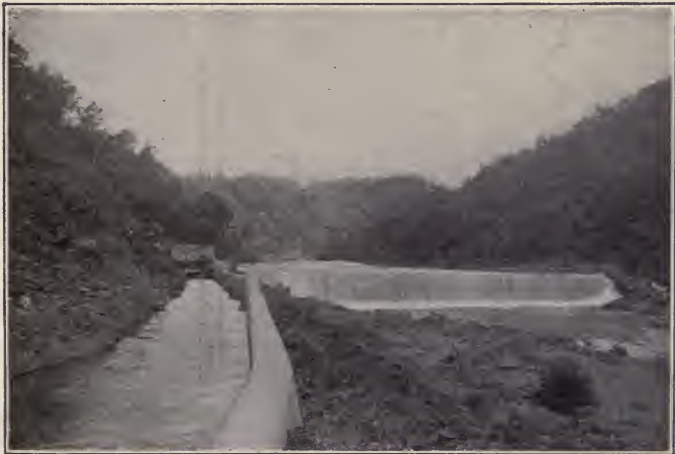
IRRIGATION DAM AND DITCH.
