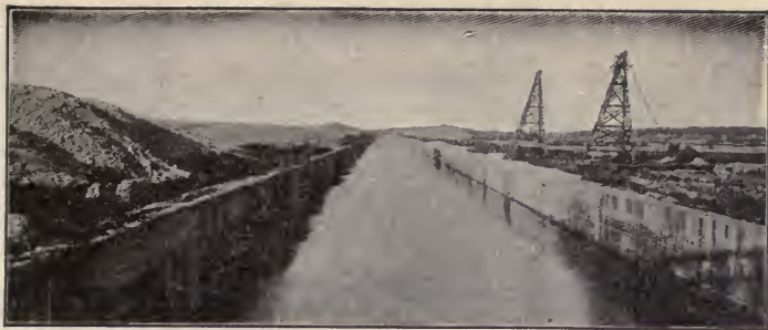
1. A section of the canal cut through solid rock.
