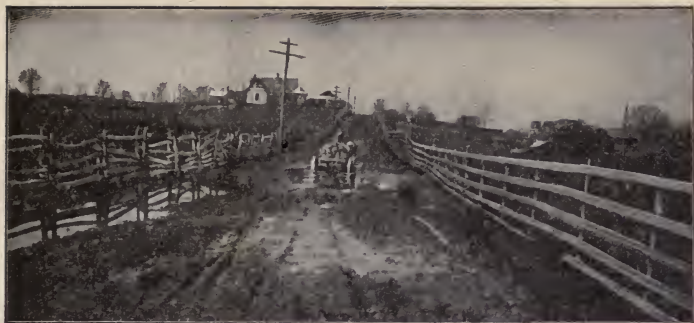
1. The road in its original condition.
