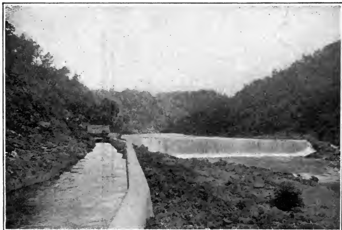
IRRIGATION DAM AND DITCH.
