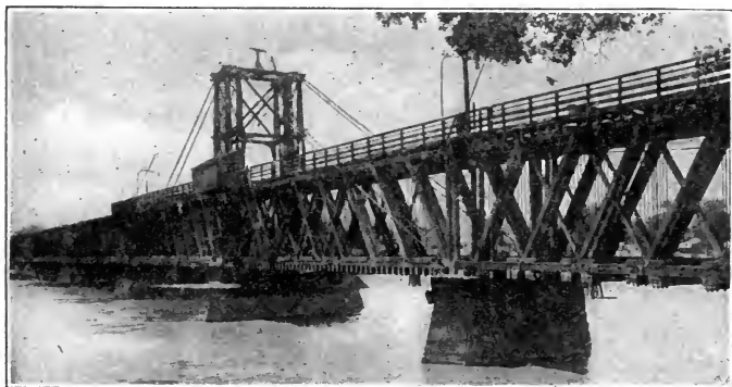
COMBINED RAILROAD AND COUNTY BRIDGE ACROSS THE SACRAMENTO RIVER, CAL.
