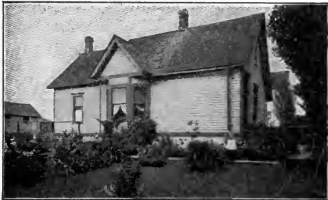
THE WELL-KEPT HOME OF AN EMPLOYEE OF A MINING COMPANY.
