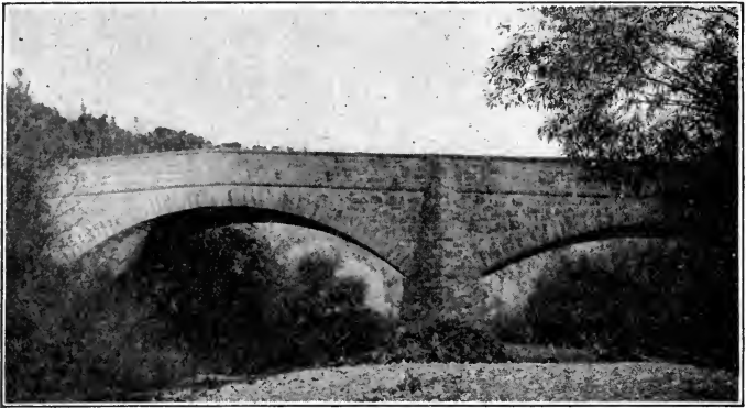
EXAMPLE OF PERMANENT ROAD WORK, NAPA COUNTY, CALIFORNIA.
