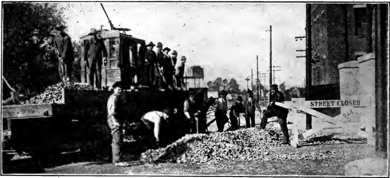
Men Repairing a Street
