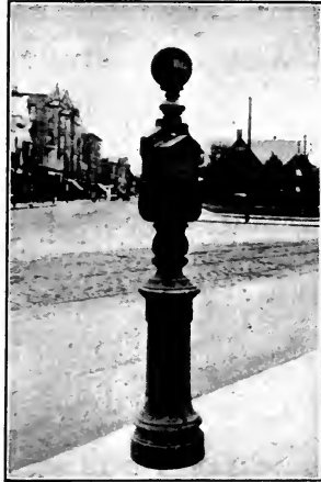
A Fire Alarm Box
