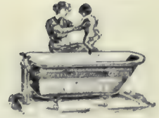
Bath Room and Lavatory Fixtures
