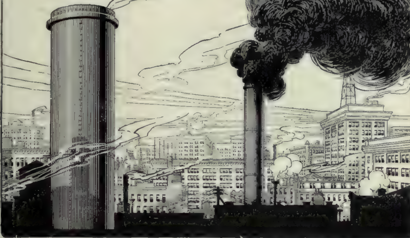
KEWANEE BOILER CHIMNEY.
