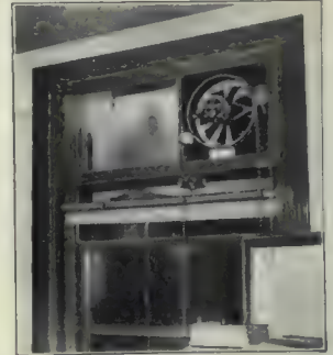
Another form of ventilation adapted to top sash of window transoms or end of skylights. The Ventura Reversible Electric Fan.
