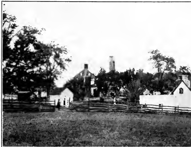
RUIN OF MUMMA'S HOUSE, ANTIETAM
