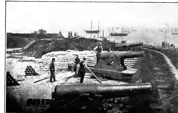
THE CONFEDERATE COMMAND OF THE RIVER. (Battery Magruder, Yorktown.) Looking north up the river, four of the five 8-inch Columbiads composing this section of the battery are visible. The grape-shot and spherical shells, which had been gathered in quantities to prevent the Federal fleet from passing up the river, were abandoned on the hasty retreat of the Confederates, the guns being spiked. The vessels in the river are transport ships, with the exception of the frigate just off shore.
