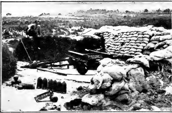
RAMPARTS THAT BAFLED McCLELLAN. (Hasty fortifications of the Confederates at Yorktown.) It was against such fortifications as these, which Magruder had hastily reenforced with sand-bags, that McClellan spent a month preparing his heavy batteries. Magruder had far too few soldiers to man his long line of defenses properly, and his position could have been taken by a single determined attack. This rampart was occupied by the Confederate general, D. H. Hill, who had been the first to enter Yorktown in order to prepare it for siege. He was the last to leave it on the night of May 3, 1862.
