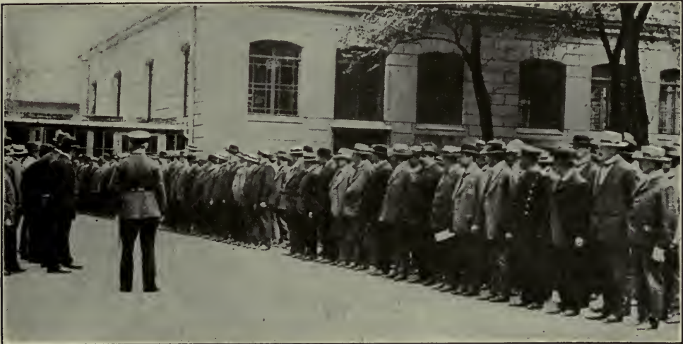
Mobilizing the Landsturm at Leipsic
