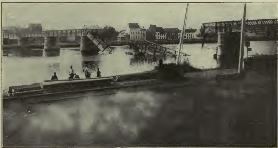
Dynamited Bridge Across the Meuse, at Vise, Belgium
