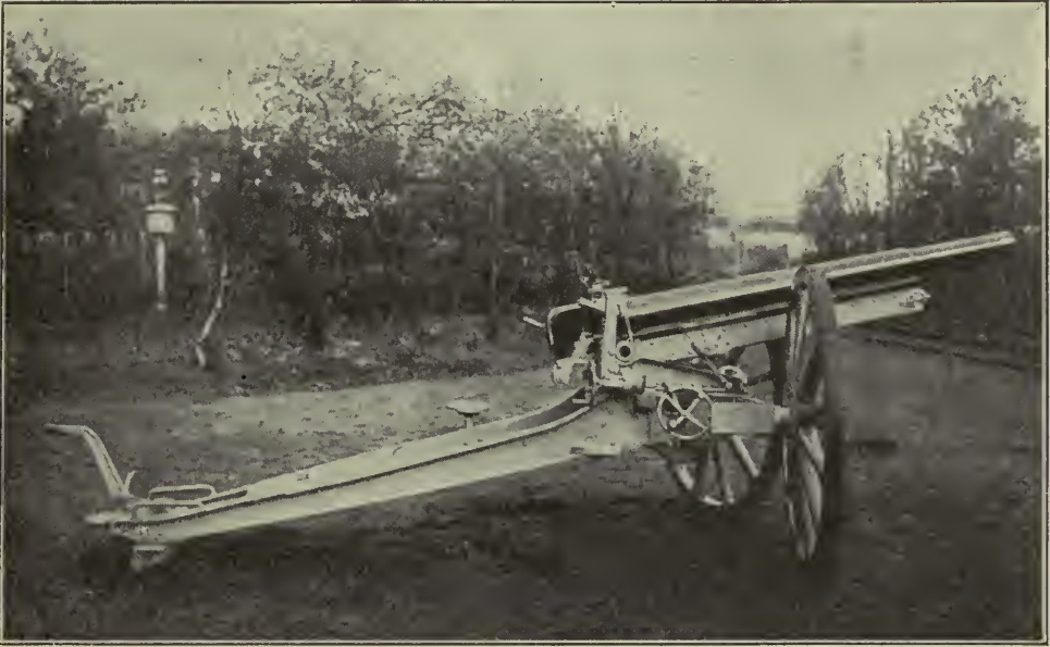
German Field Piece with Interlocking Wheels
