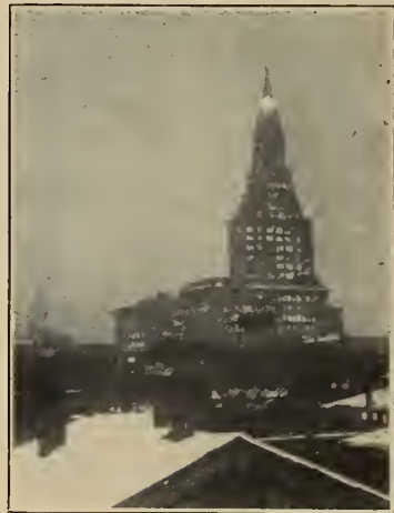
THIRD NATIONAL BANK BUILDING Springfield, Massachusetts
