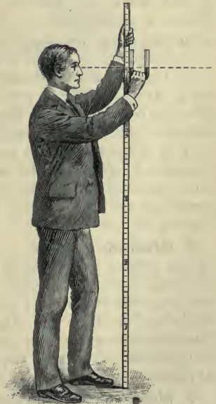
FIG. 9.—A simple water-level and levelling staff used for measuring relative heights.
