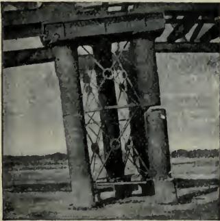
FIG. 109.—Damage done to a railway bridge at Nagara, Japan, during the great earthquake of October, 1891.
