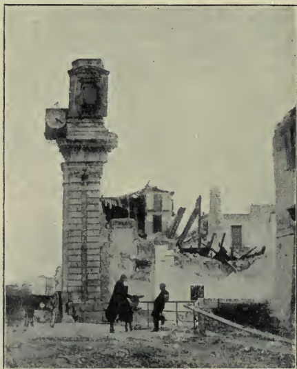
FIG. 110.—Messina-Reggio earthquake of December 28, 1908. A wrecked house on Via Porta Imperiale, Messina. The clock on the corner post indicates the time of occurrence of the earthquake, 5.20 a.m. (From the Bulletin of the Imperial Earthquake Investigation Committee, Tokyo, November, 1909. )
